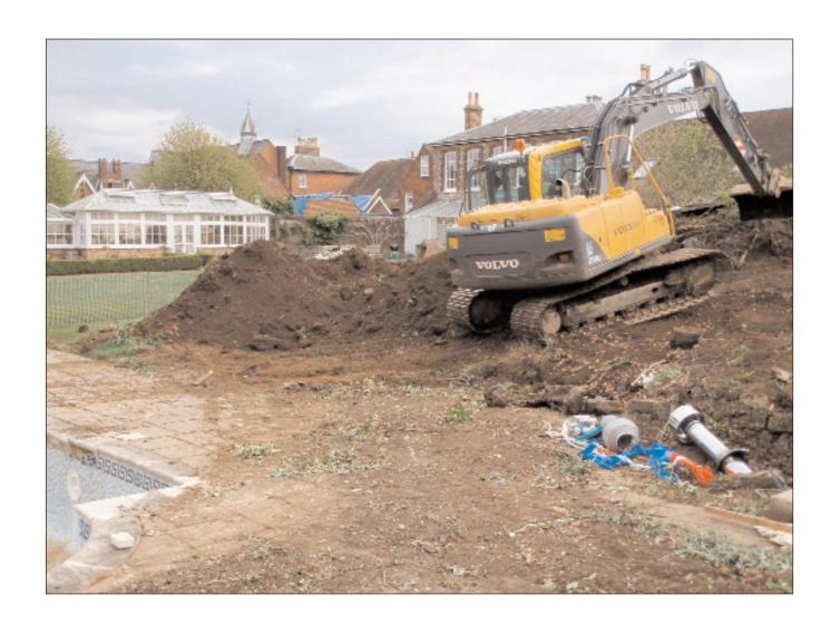
Plate 1. Topsoil stripping of site in progress by the pool (facing north).
