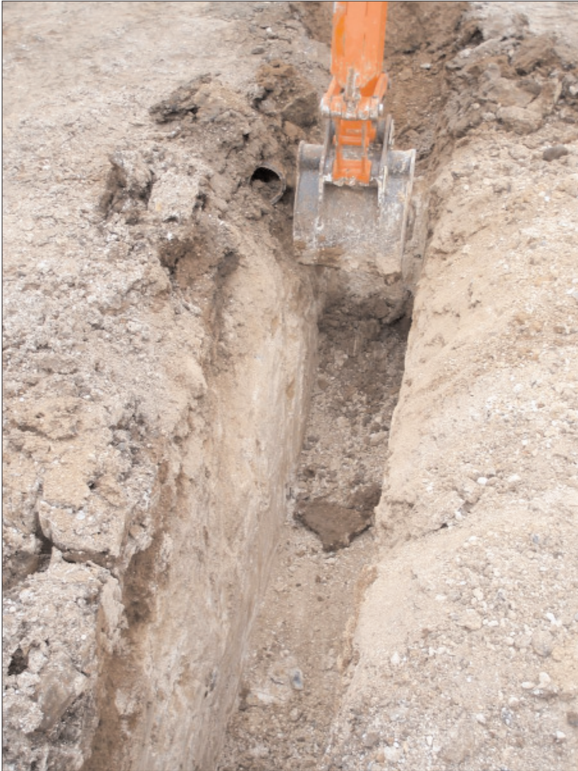
Plate 2. Foundation trench cut (Looking south-east).
