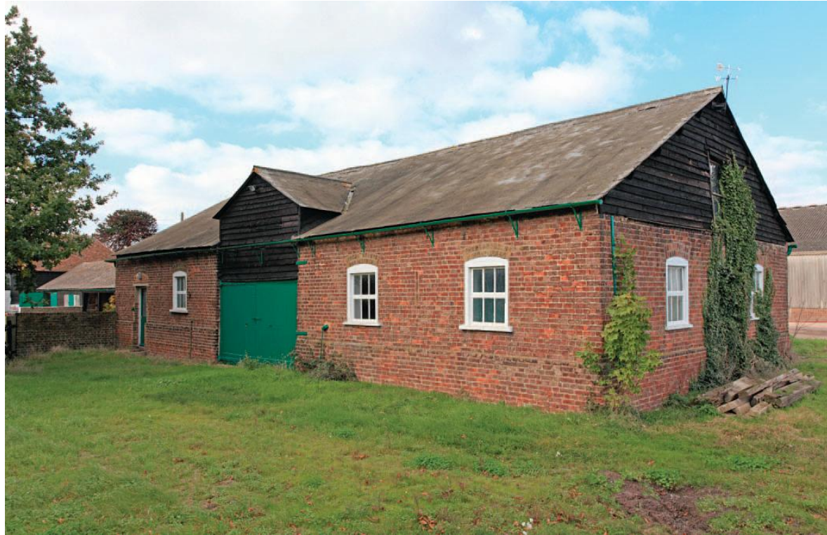
Plate 3 Court Lodge Farm. Barn Building to be converted in to Residential Property. Facing North.
