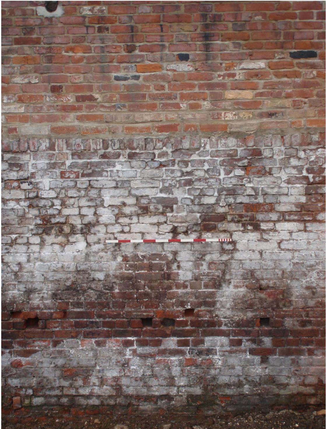
**Plate 11. Section of wall [W03 & W05]. Note holes for benches**
