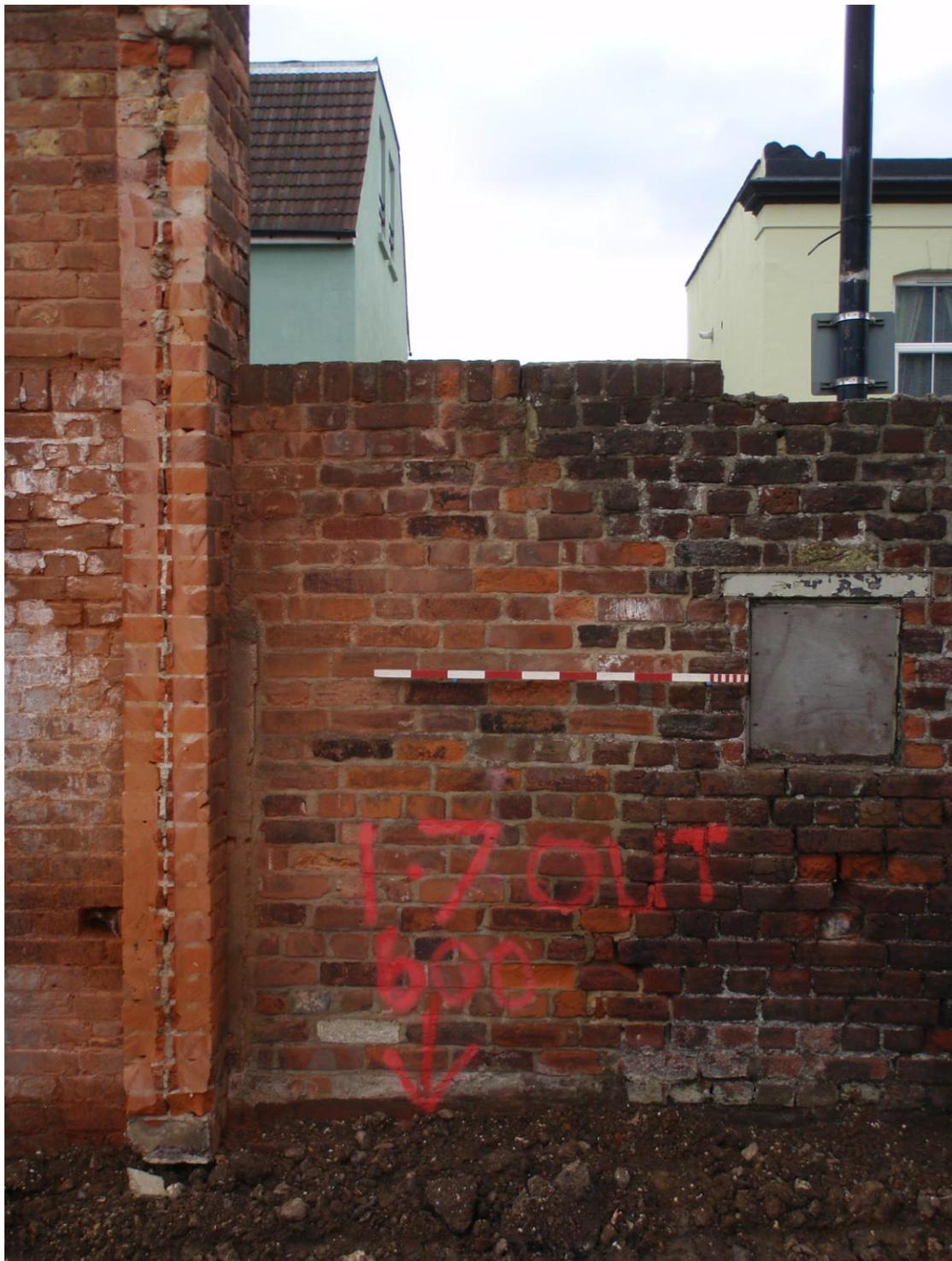
Plate 12. Section of wall showing small window and brick repair [W04, W07]
