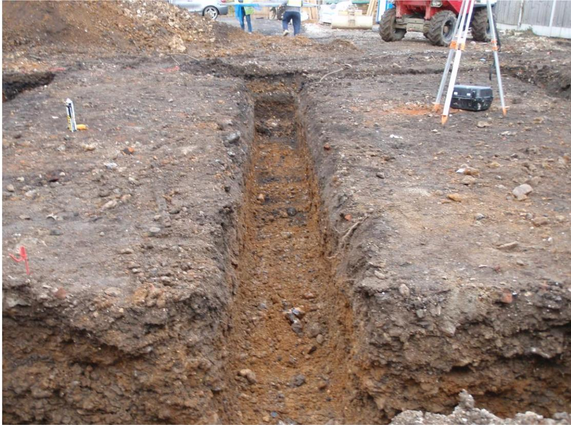
Plate 14. Foundation trenches for new development
