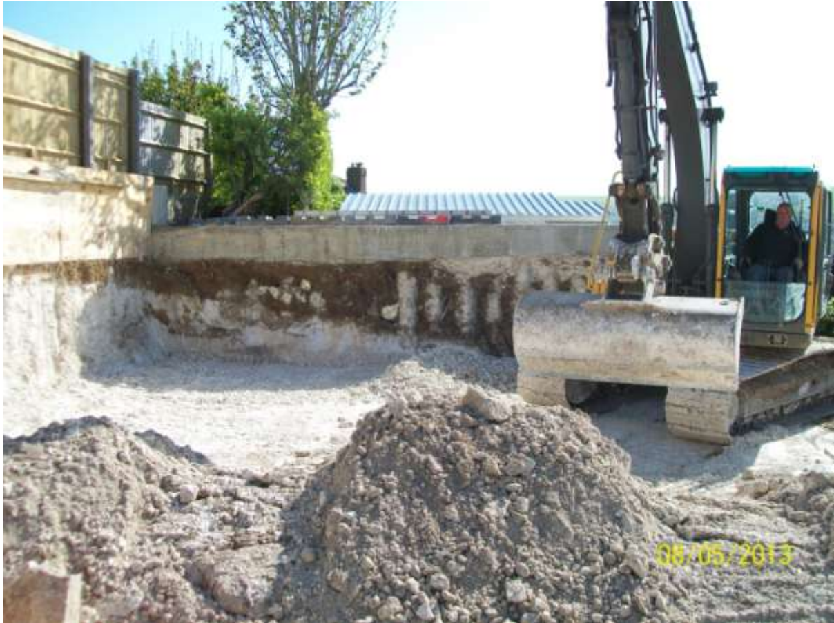
Plate 6. Area strip of topsoil and chalk showing site piling exposed to the east (facing east)
