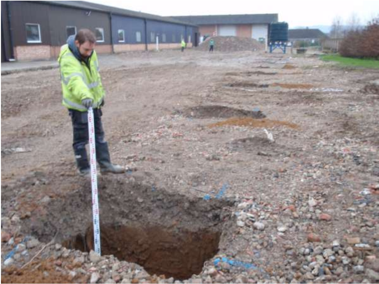
Plate 3. The site showing ground works (post pads) facing south
