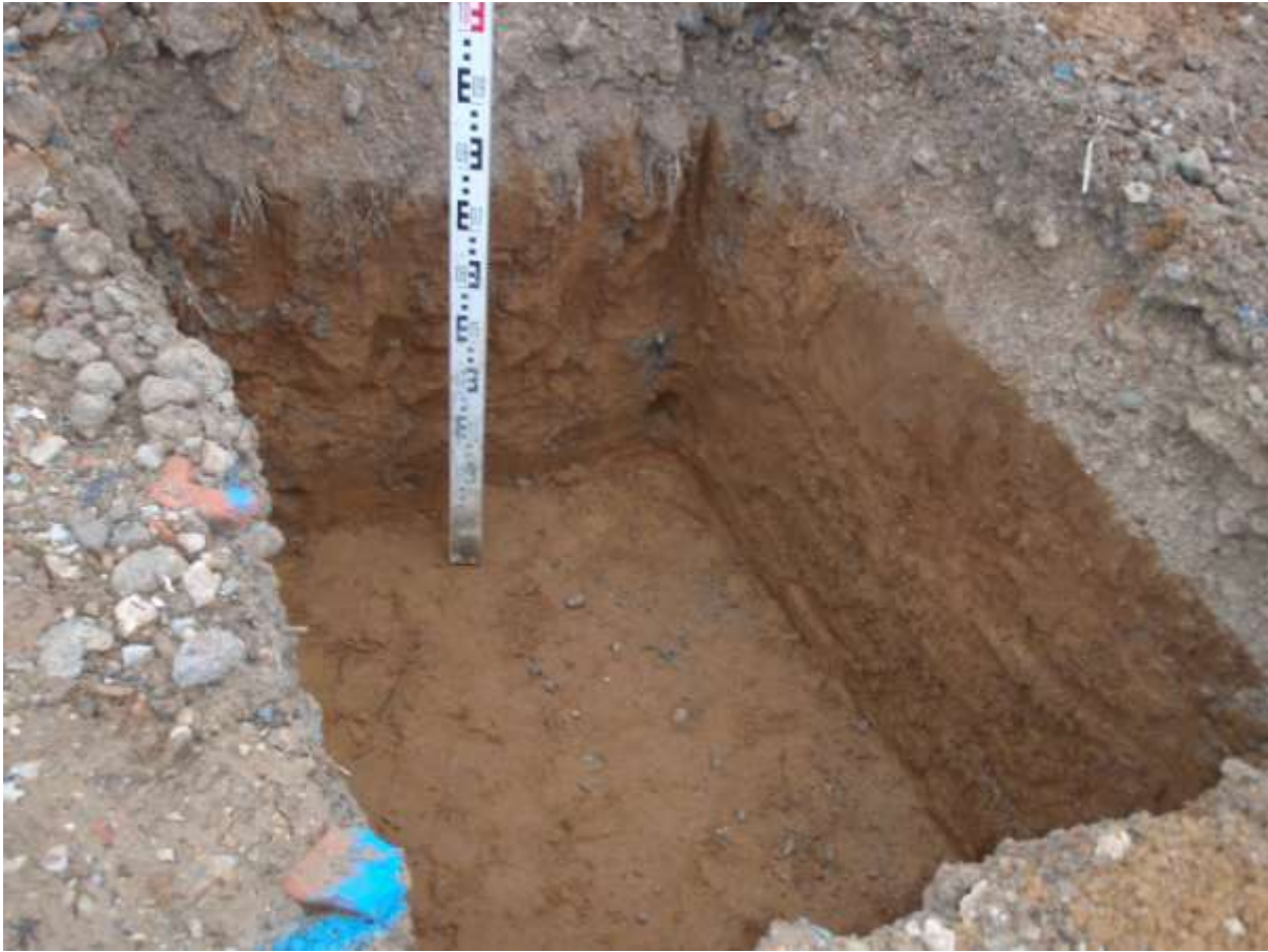
Plate 4. Foundation pad showing geology (facing north)
