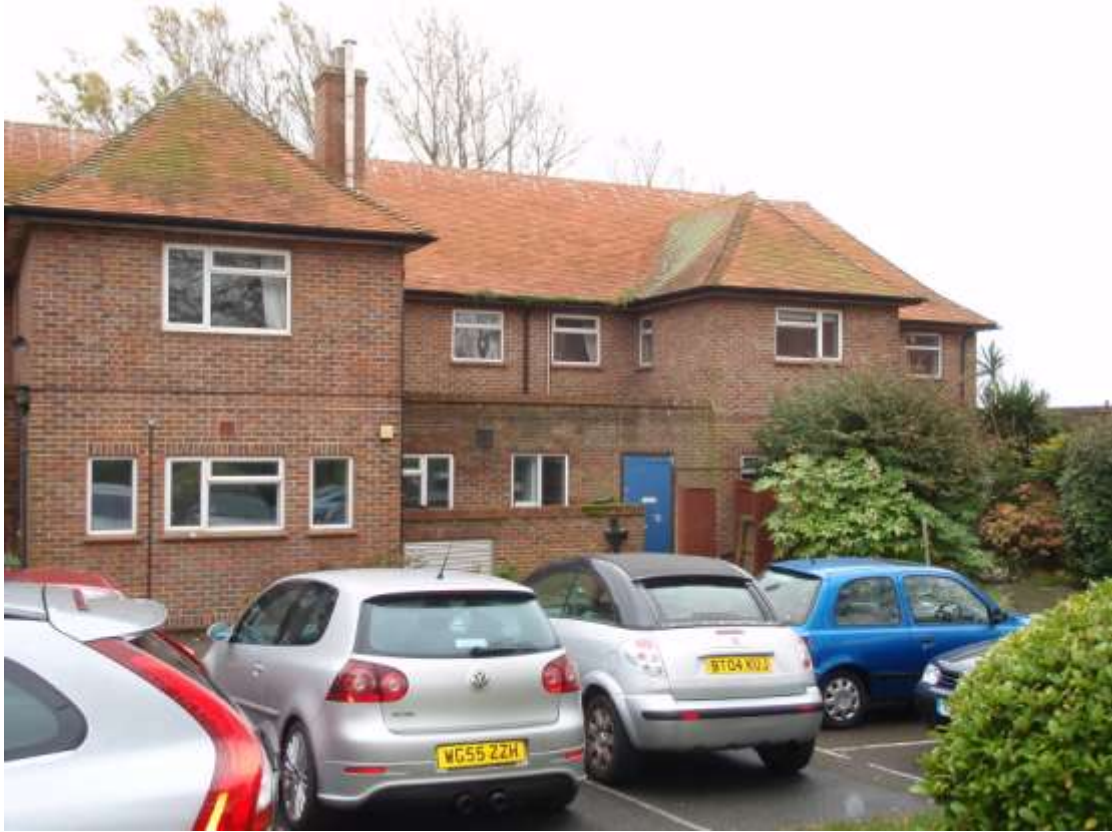
Plate 2. Development site, buildings to be demolished, facing south
