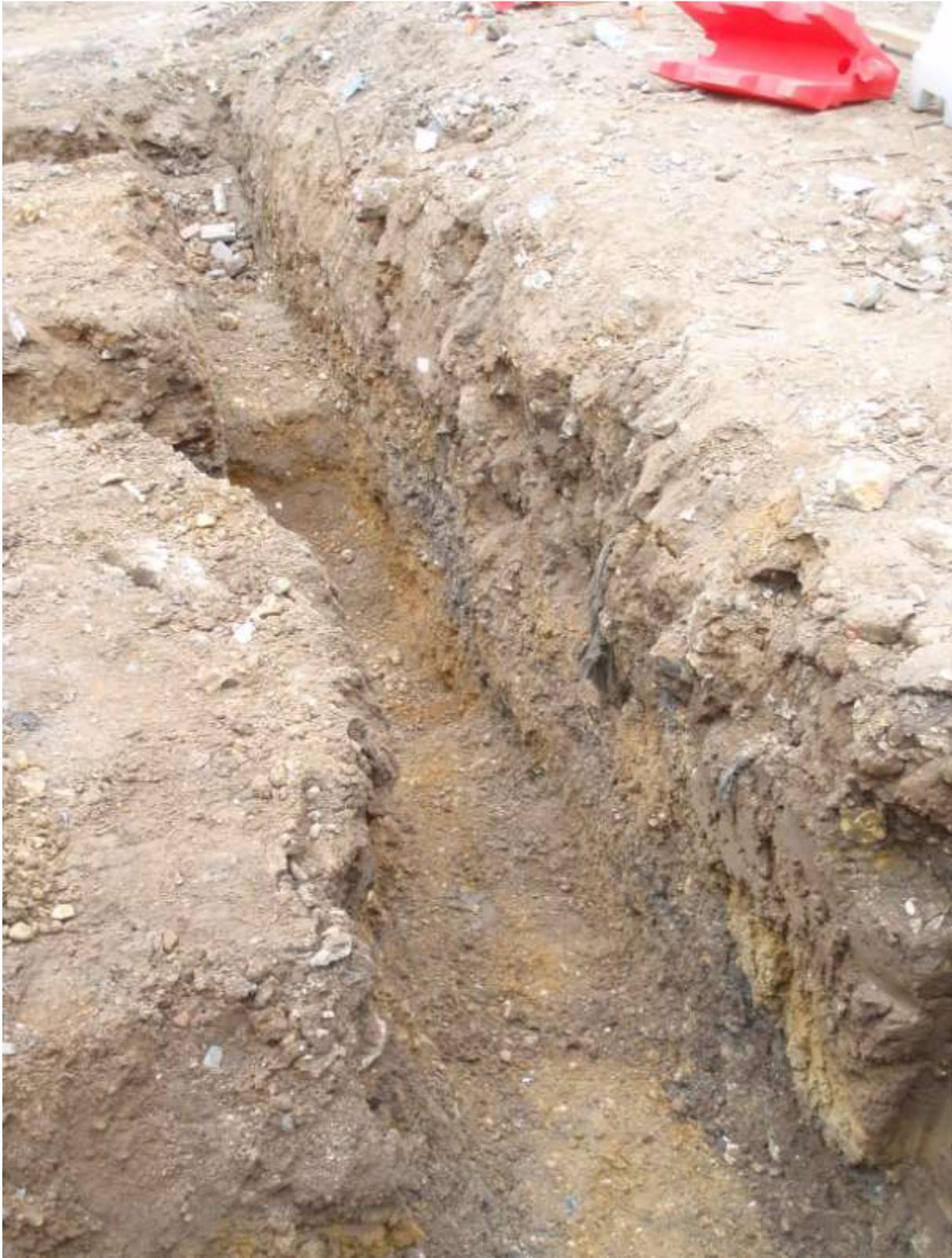
**Plate 4. Foundation trench showing geology (facing north)**
