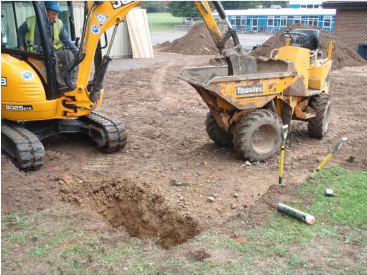
Plate 3. The site showing cutting of foundation trenches (facing north-east)
