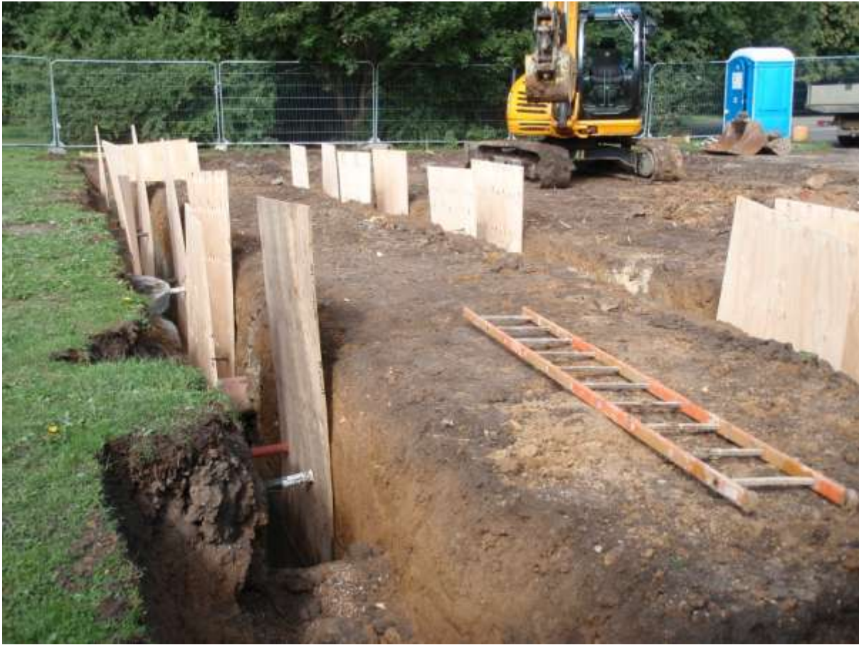
Plate 4. Foundation trenches (facing west)
