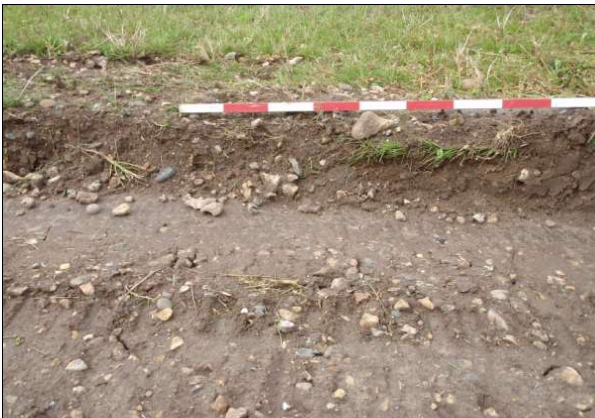
Plate 6. View of the storage compound depth of strip- 150mm (looking south-west)
