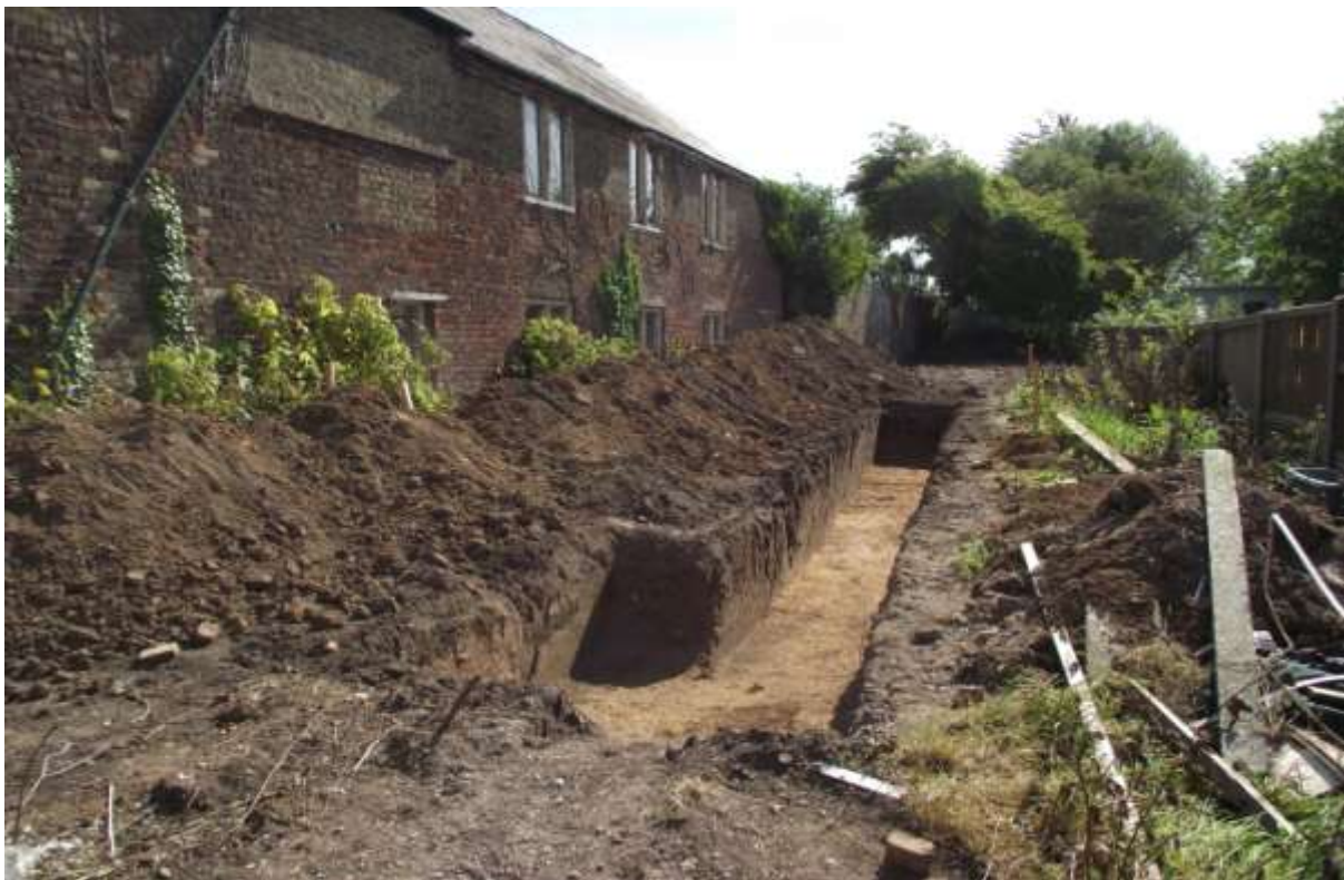
Plate 2 – Location shot of trench, looking northeast.
