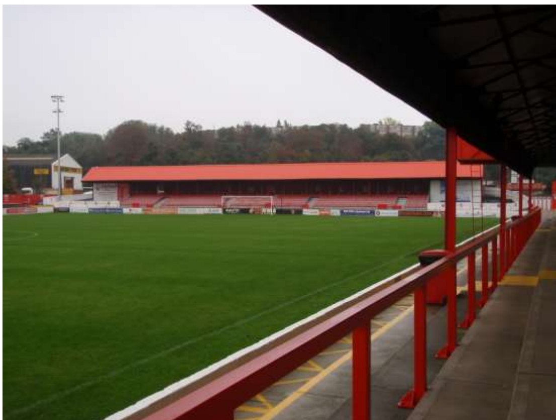
Plate 11. Looking south to the south stand
