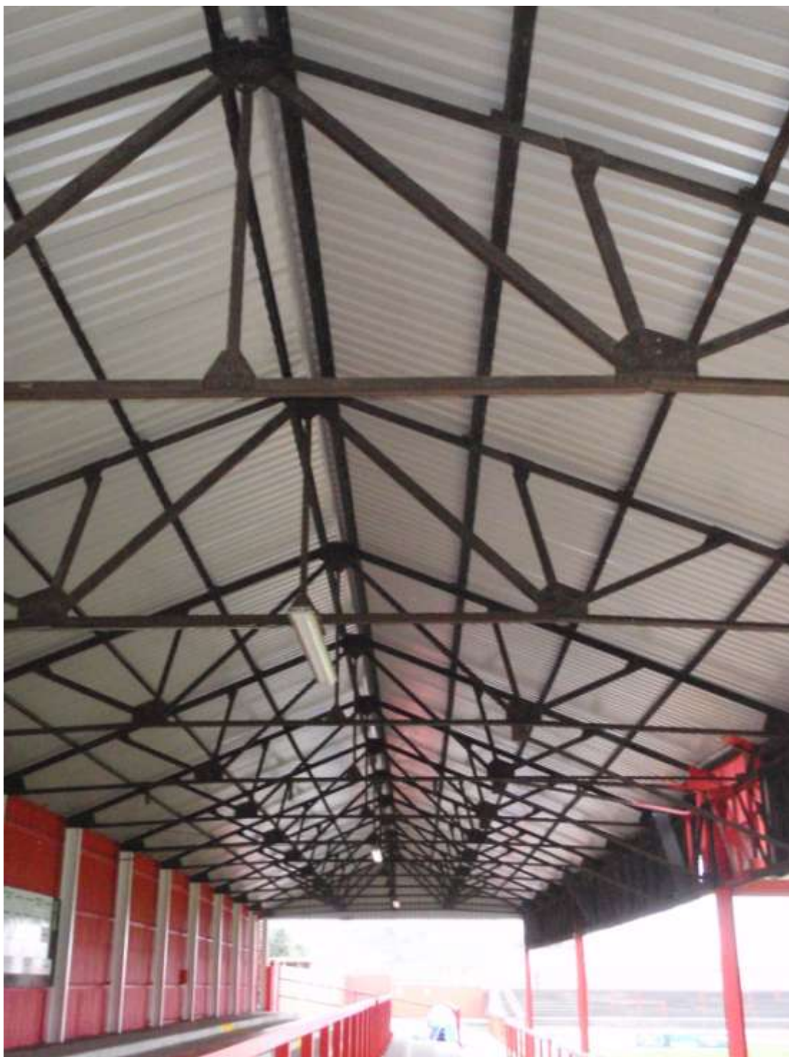
Plate 9. Inside the south-west stand showing details of roof
