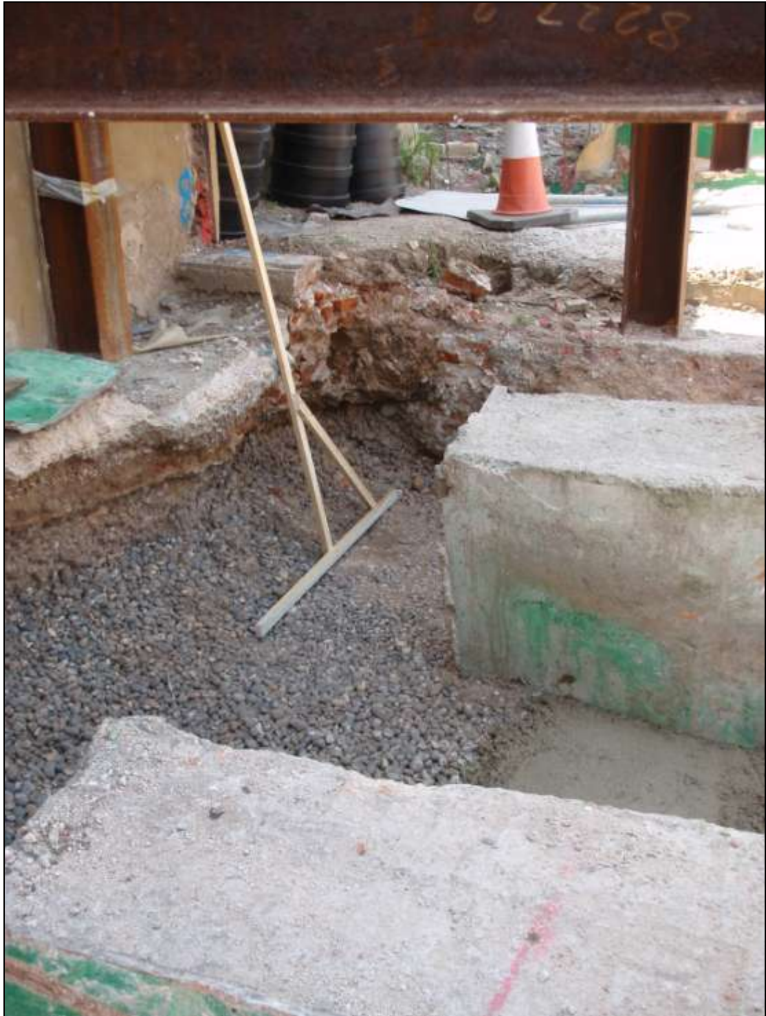
Plate 3. View of site reduction showing modern slab foundations sitting on Storm Beach Deposits (looking south-west)
