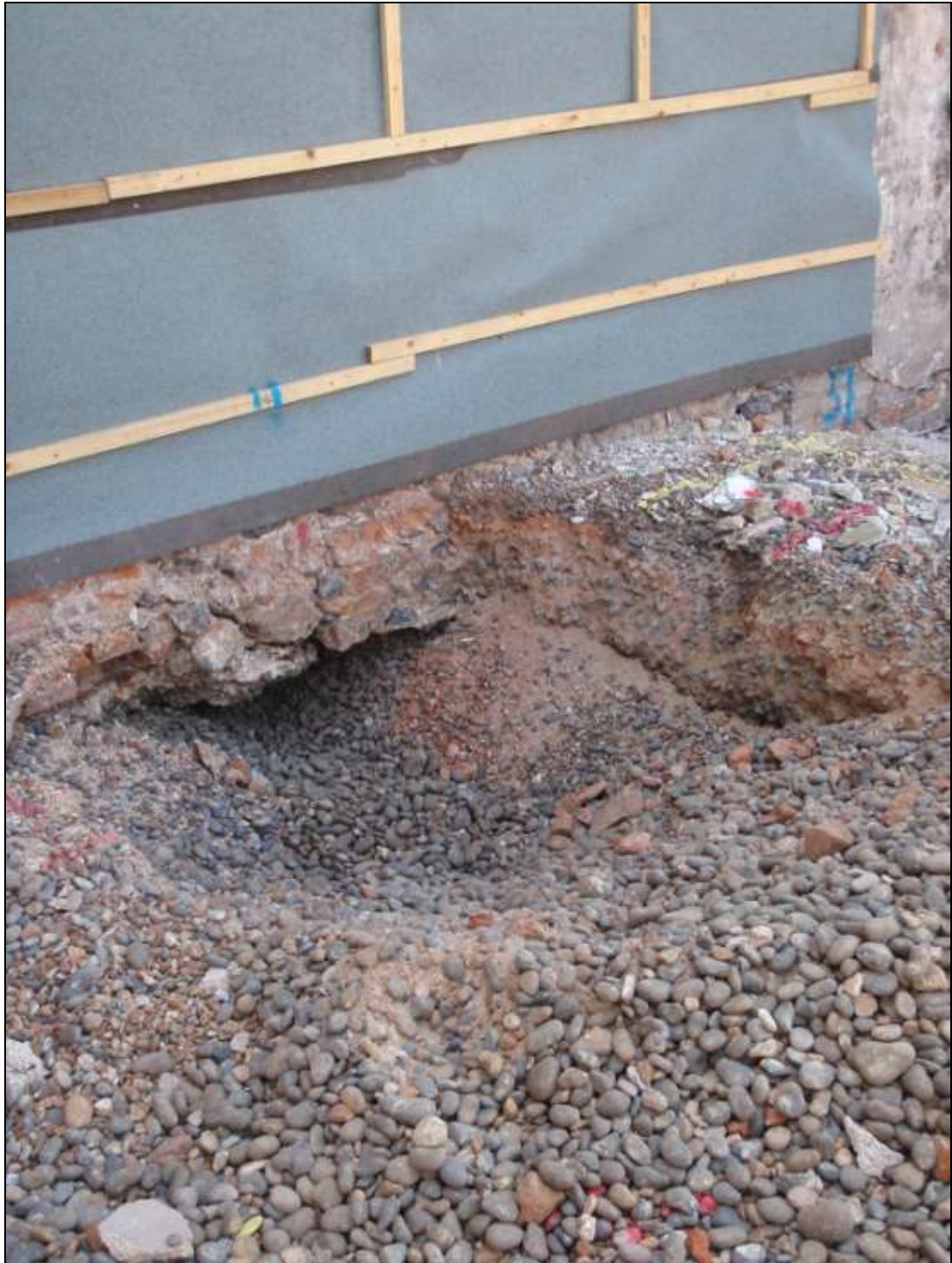
Plate 4. View of site reduction showing Storm Beach Deposits and shallow foundations of adjoining property (looking south)
