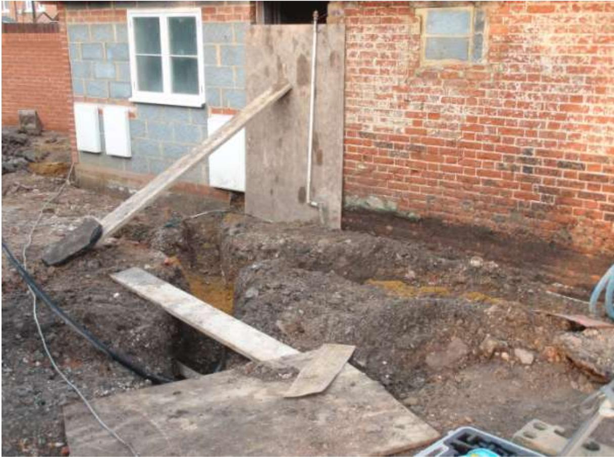
**Plate 5. Utility trenching in made-up ground**
