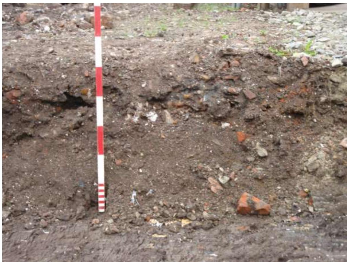
**Plate 3. The site showing the made-up ground in foundation trenches for ring beam (facing west)**
