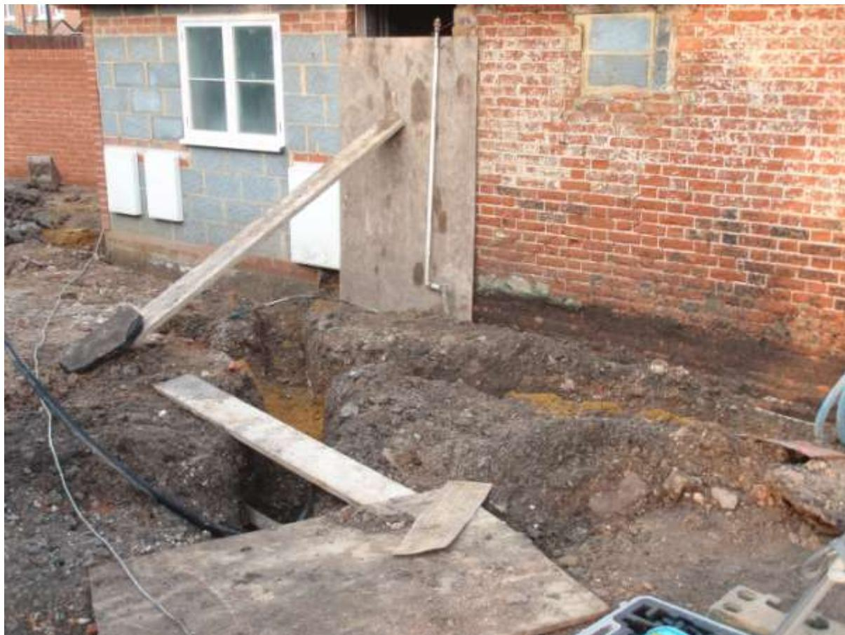
**Plate 5. Utility trenching in made-up ground**
