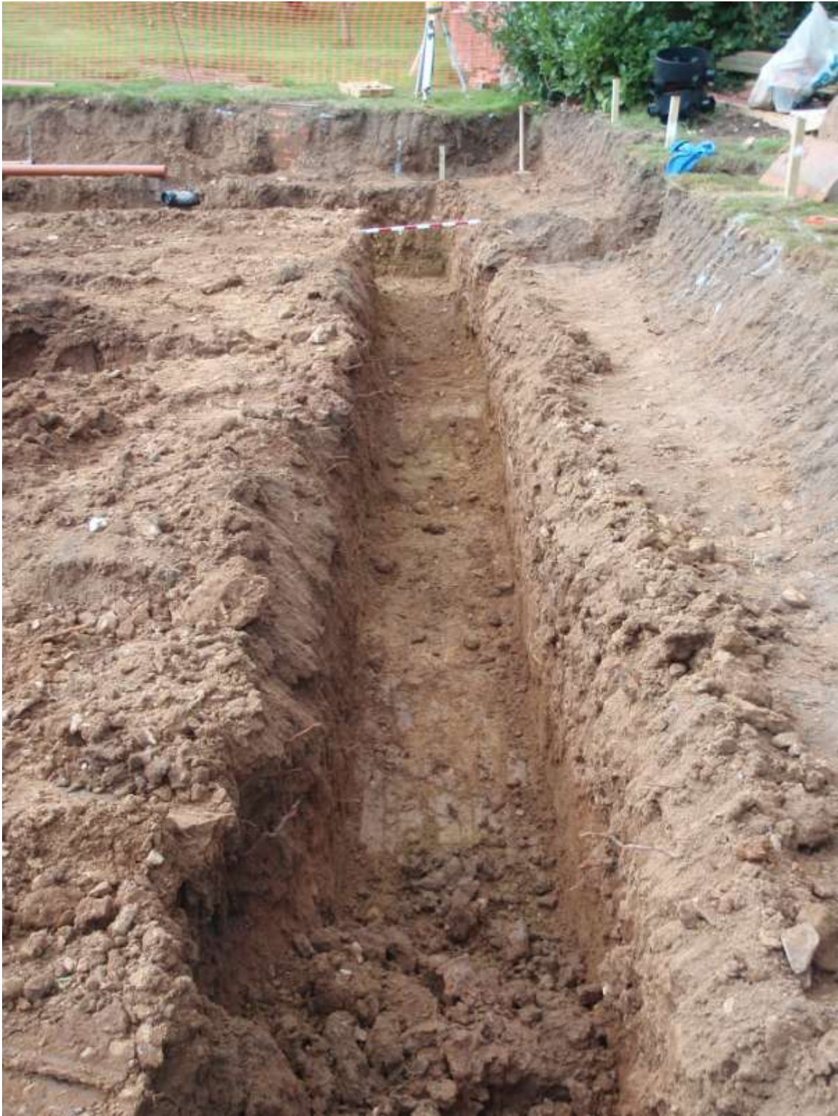
Plate 4. Trenches being excavated (looking south)
