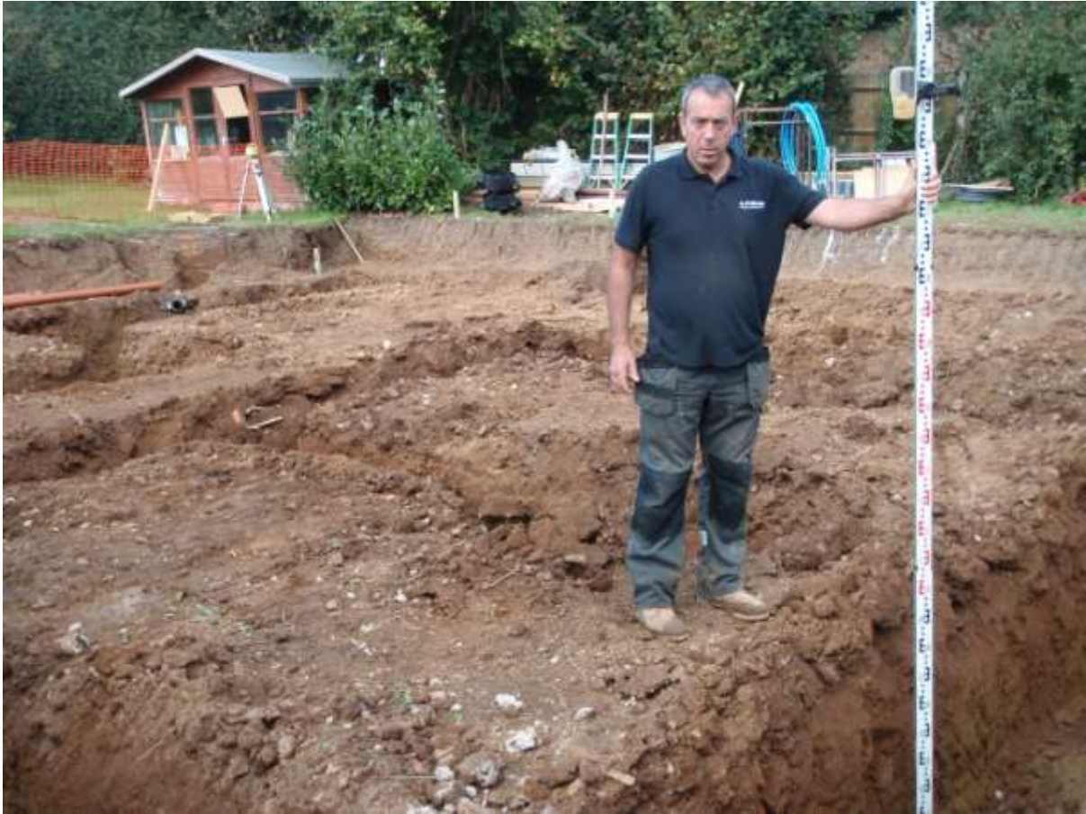
Plate 2. View of the site after topsoil strip and cutting trenches (looking north-east)
