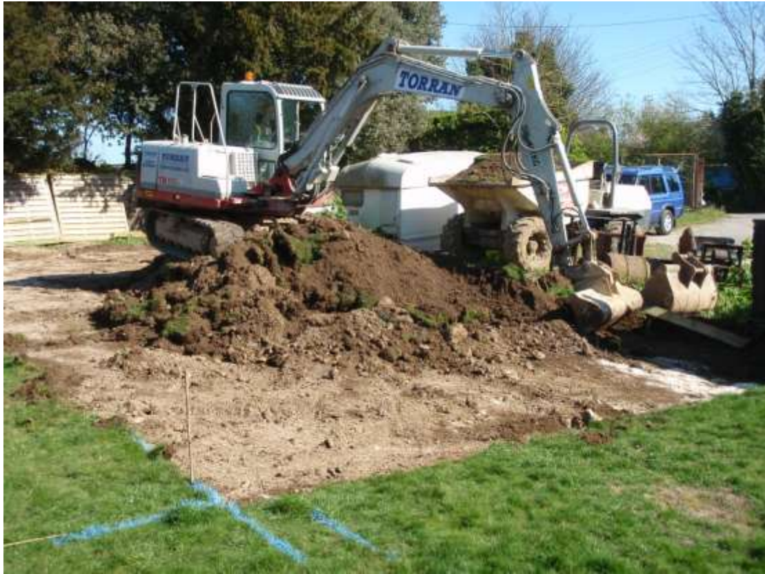
Plate 3. View of topsoil strip (looking north-east)
