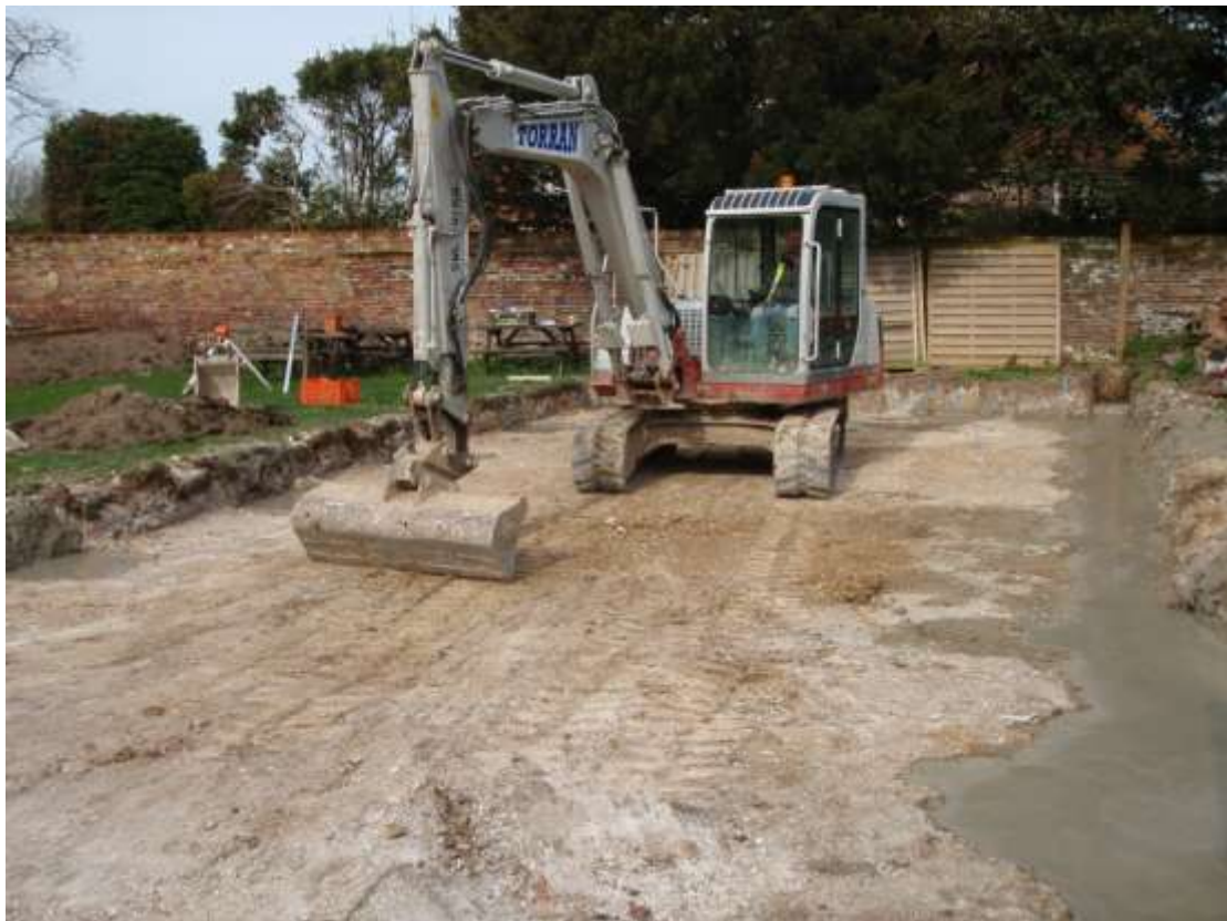
Plate 4. View of ground reduction (looking north-west)
