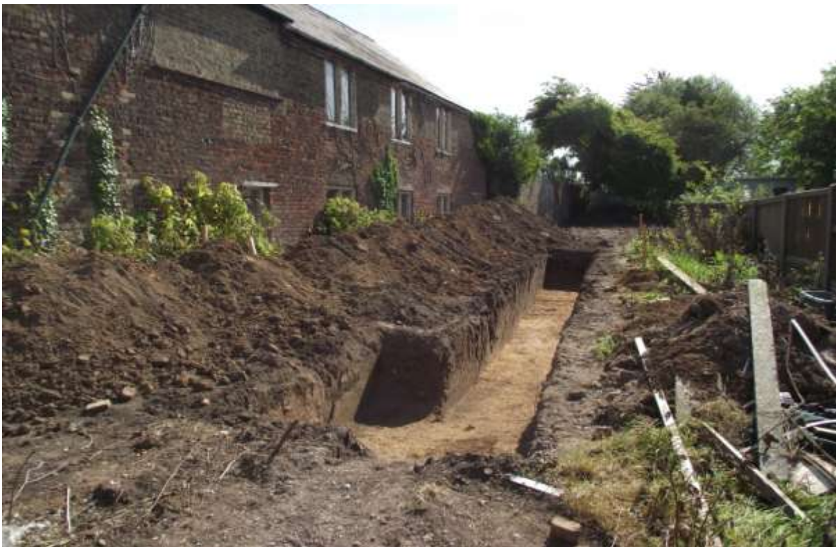
Plate 2 – Location shot of trench, looking northeast.
