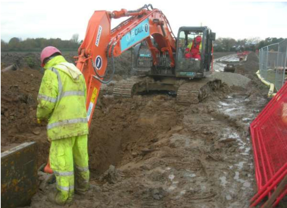
Plate 4. Phase 1. Topsoil strip. Plate 5 (below) Phase 2. Cutting trench for pipe
