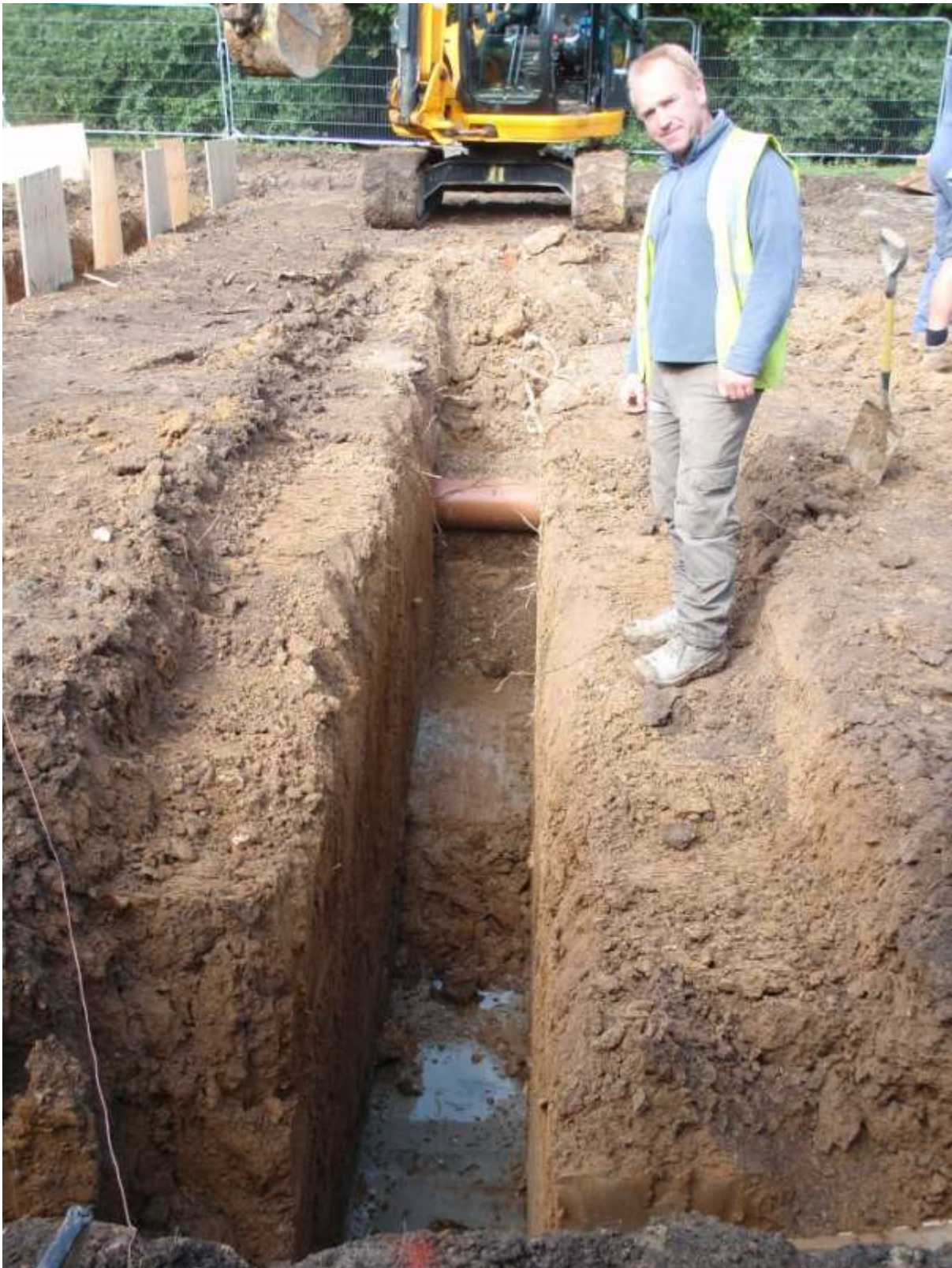
Plate 2. The site showing cutting of foundation trenches (facing north-west)
