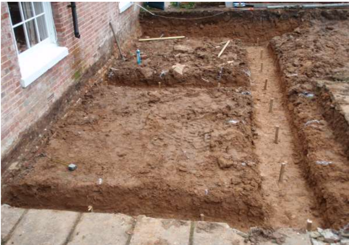
Plate 5. The site showing all foundations cut
