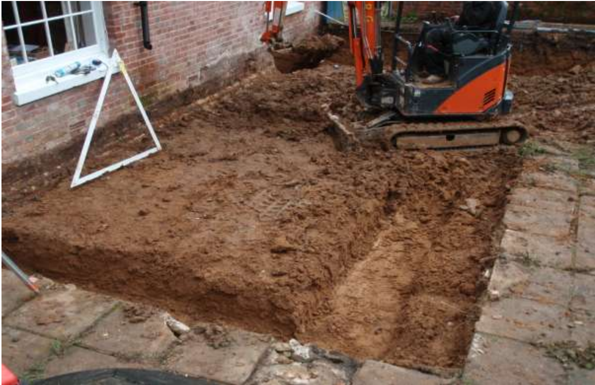
Plate 4. The site showing cutting of foundation trenches
