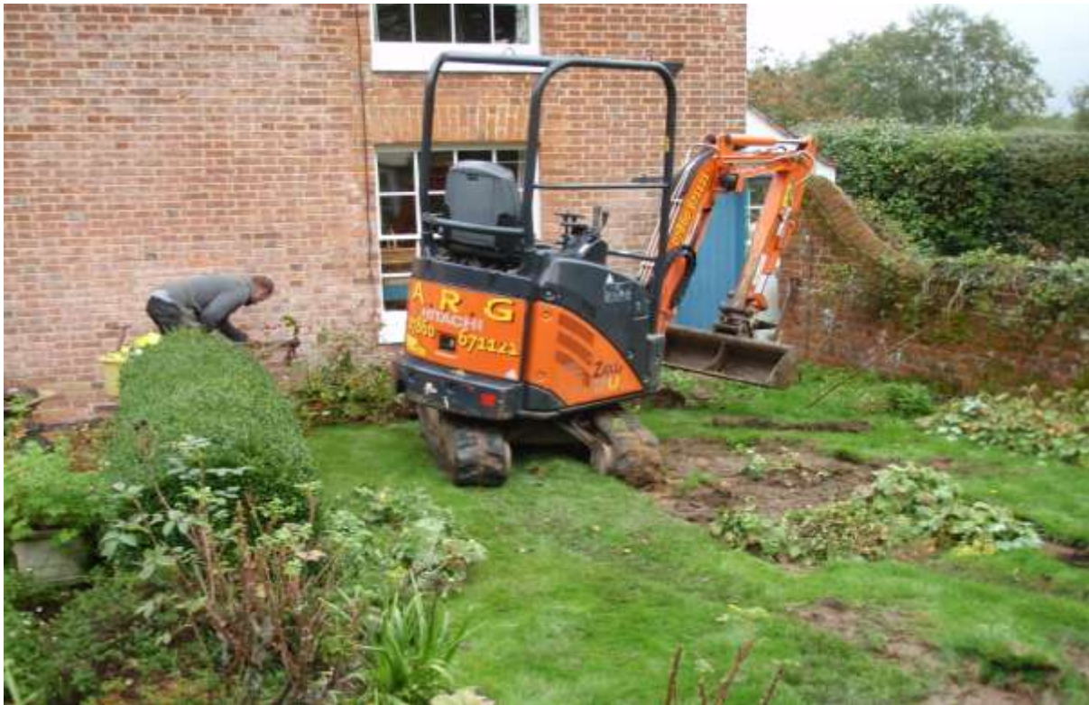
Plate 2. General view of site
