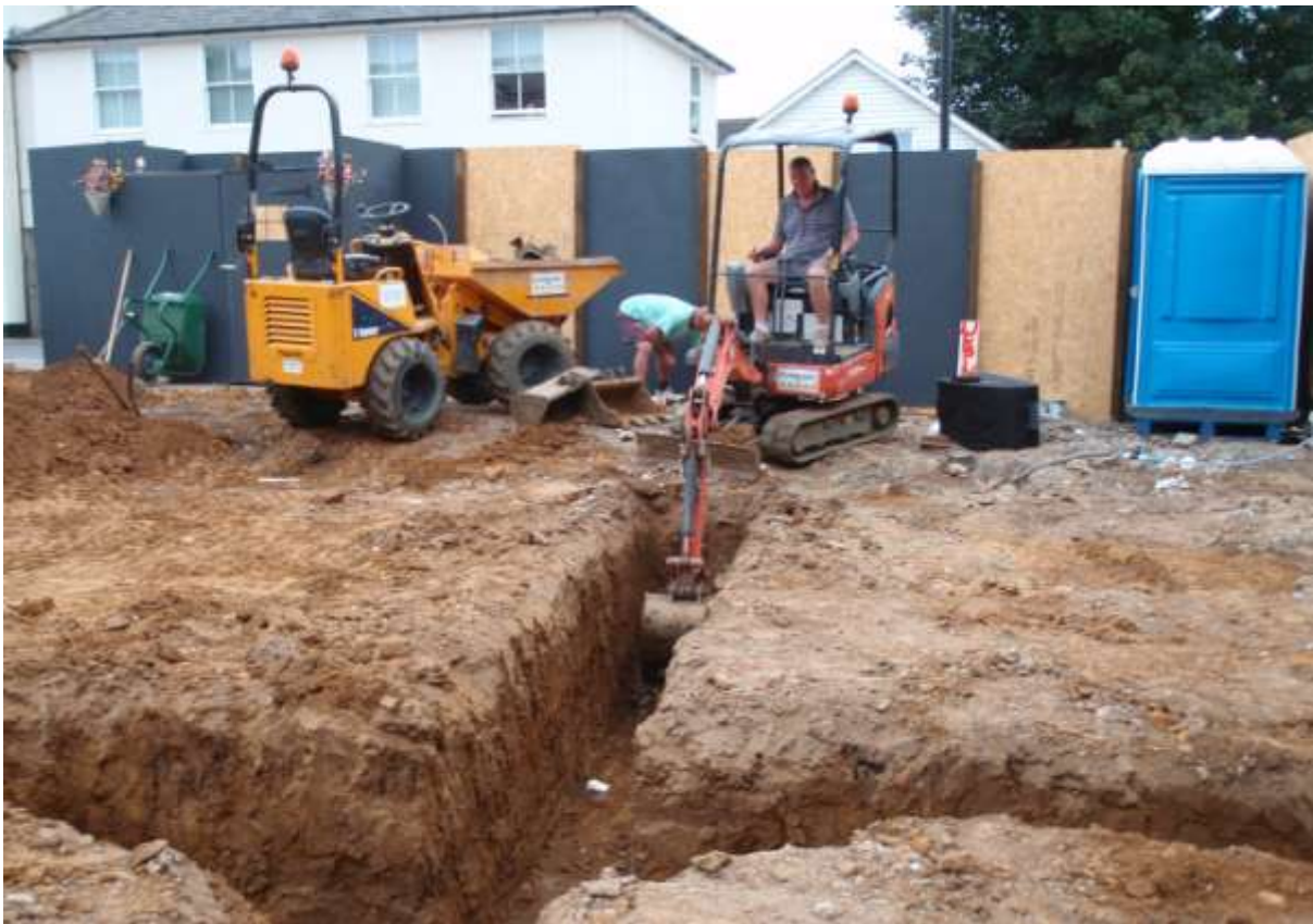
Plate 6. Cutting service trenches (facing east)
