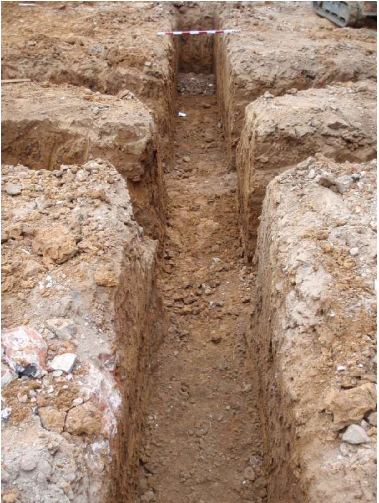
Plate 4. The site showing cutting of foundation trenches
