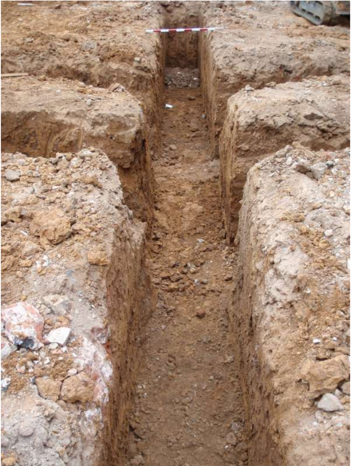
Plate 4. The site showing cutting of foundation trenches
