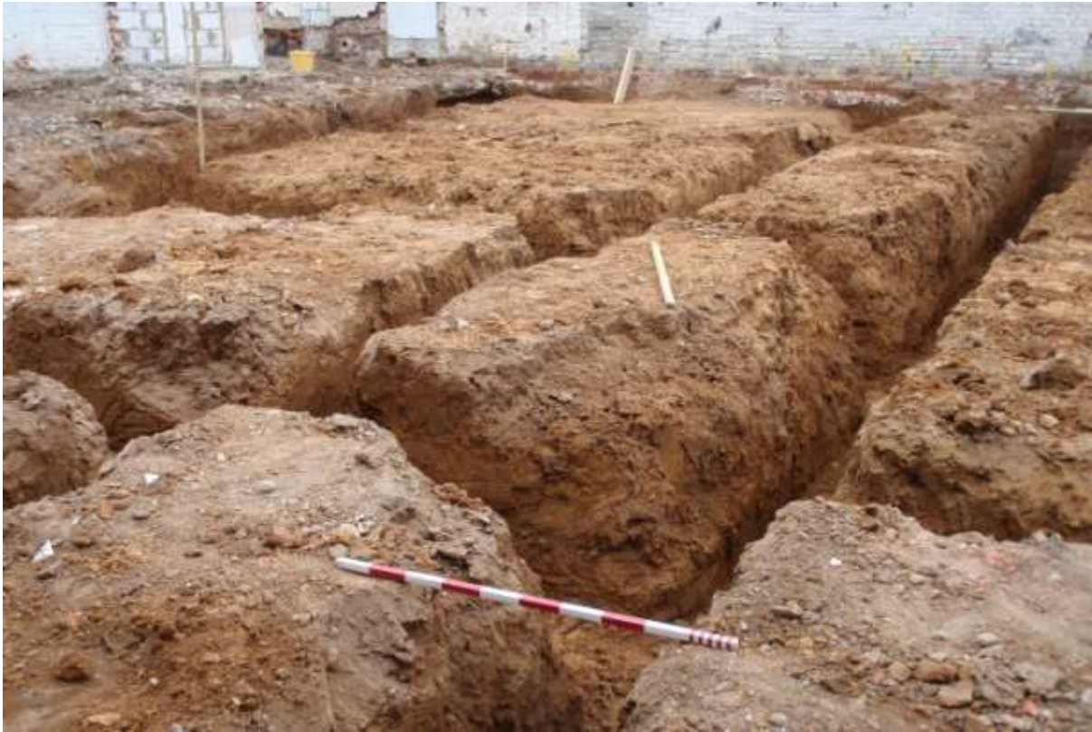
Plate 5. Foundation trenches completed
