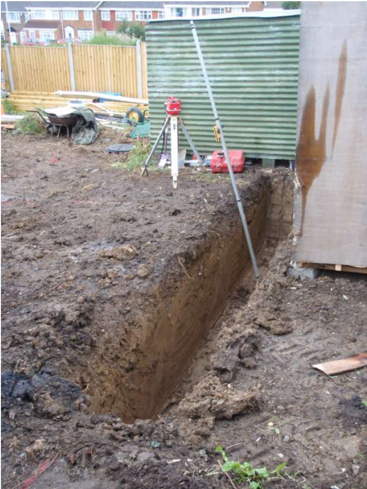
Plate 3. The site showing cutting of foundation trenches on the west side
