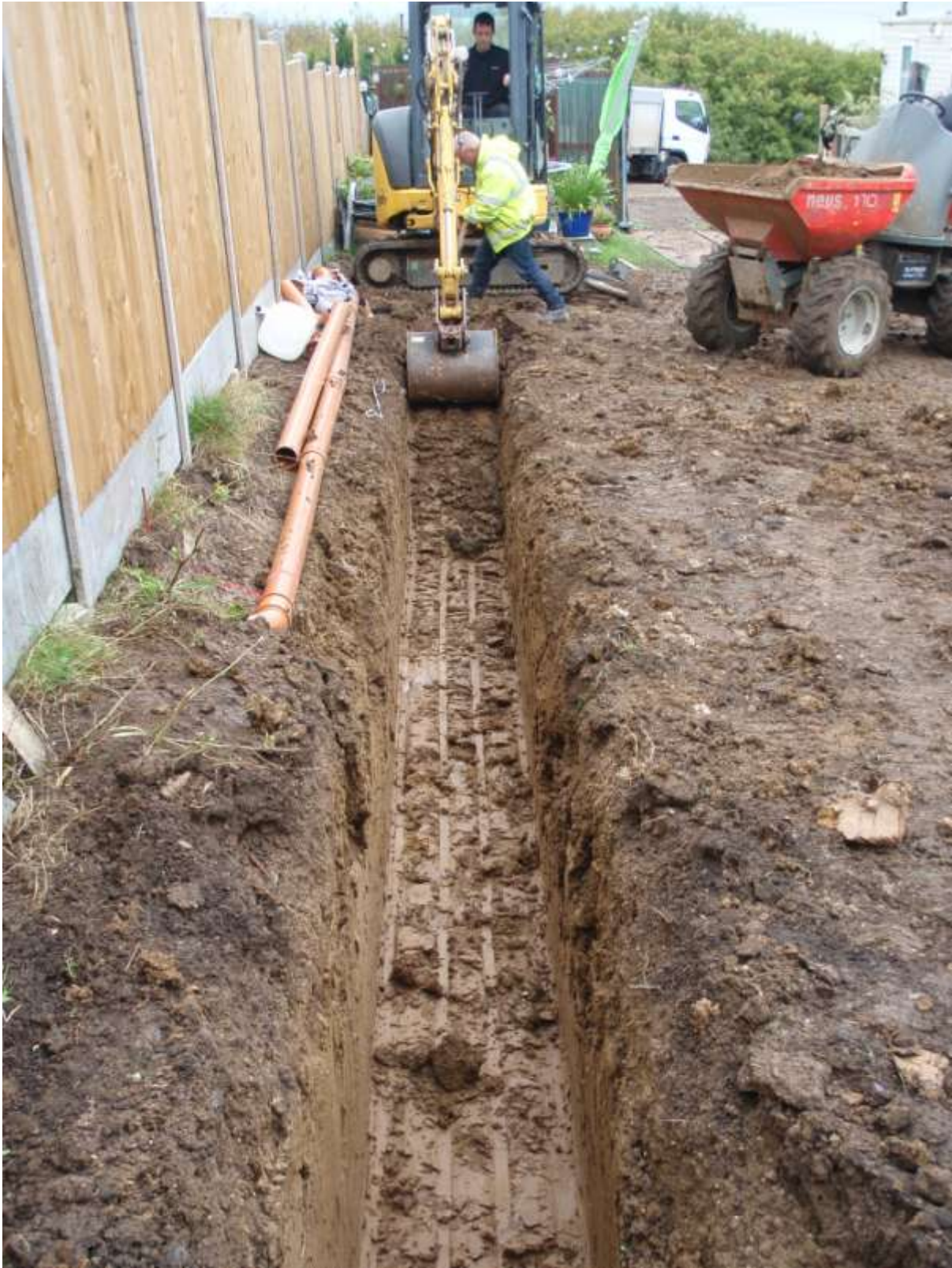
Plate 4. Foundation trenches on the north side
