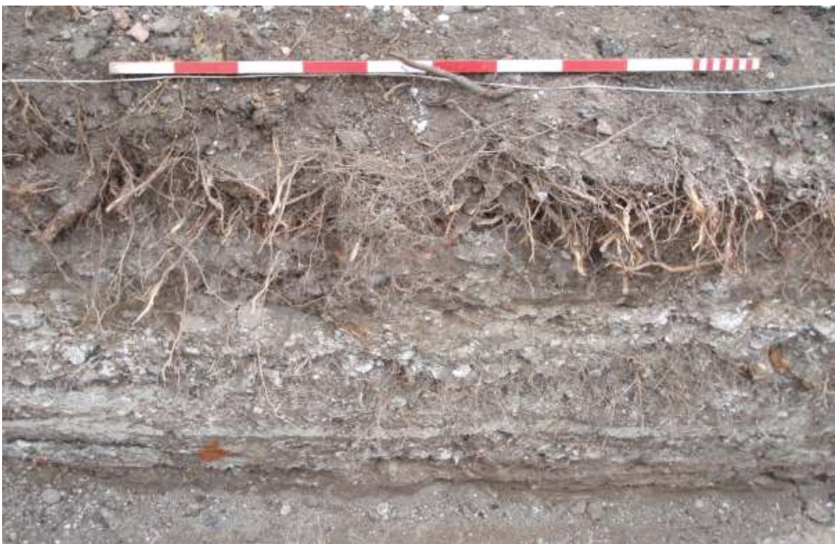
Plate 3. The site showing section of foundation trench
