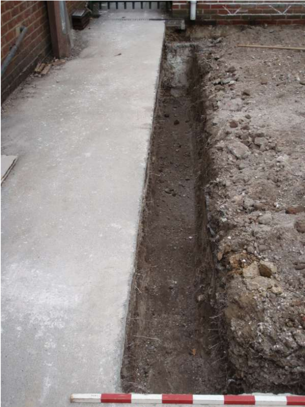
Plate 5. Foundation trenches on the south side
