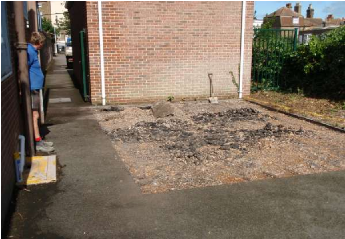
Plate 2. General view of site with tarmac removed
