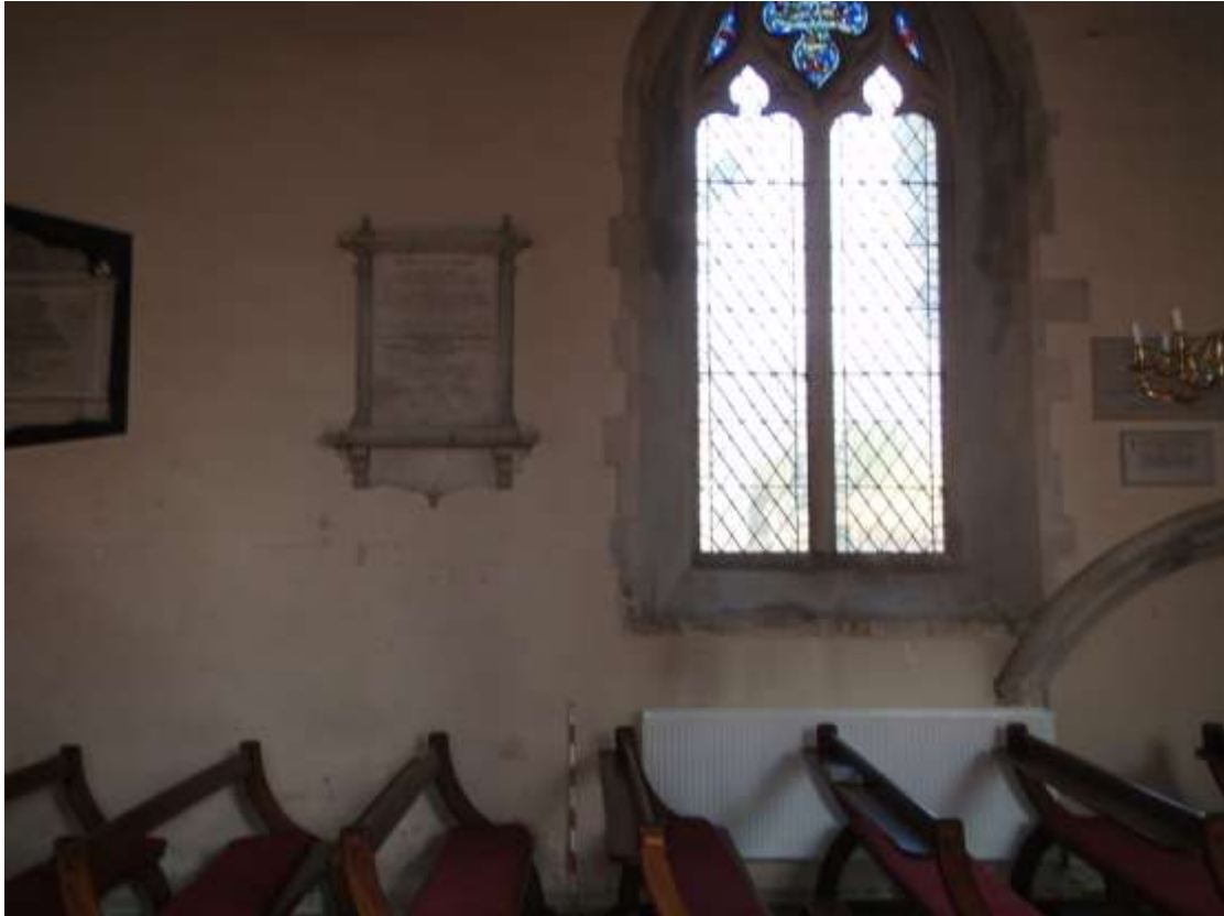
Plate 6. Proposed Development site, interior of north wall (Looking north)
