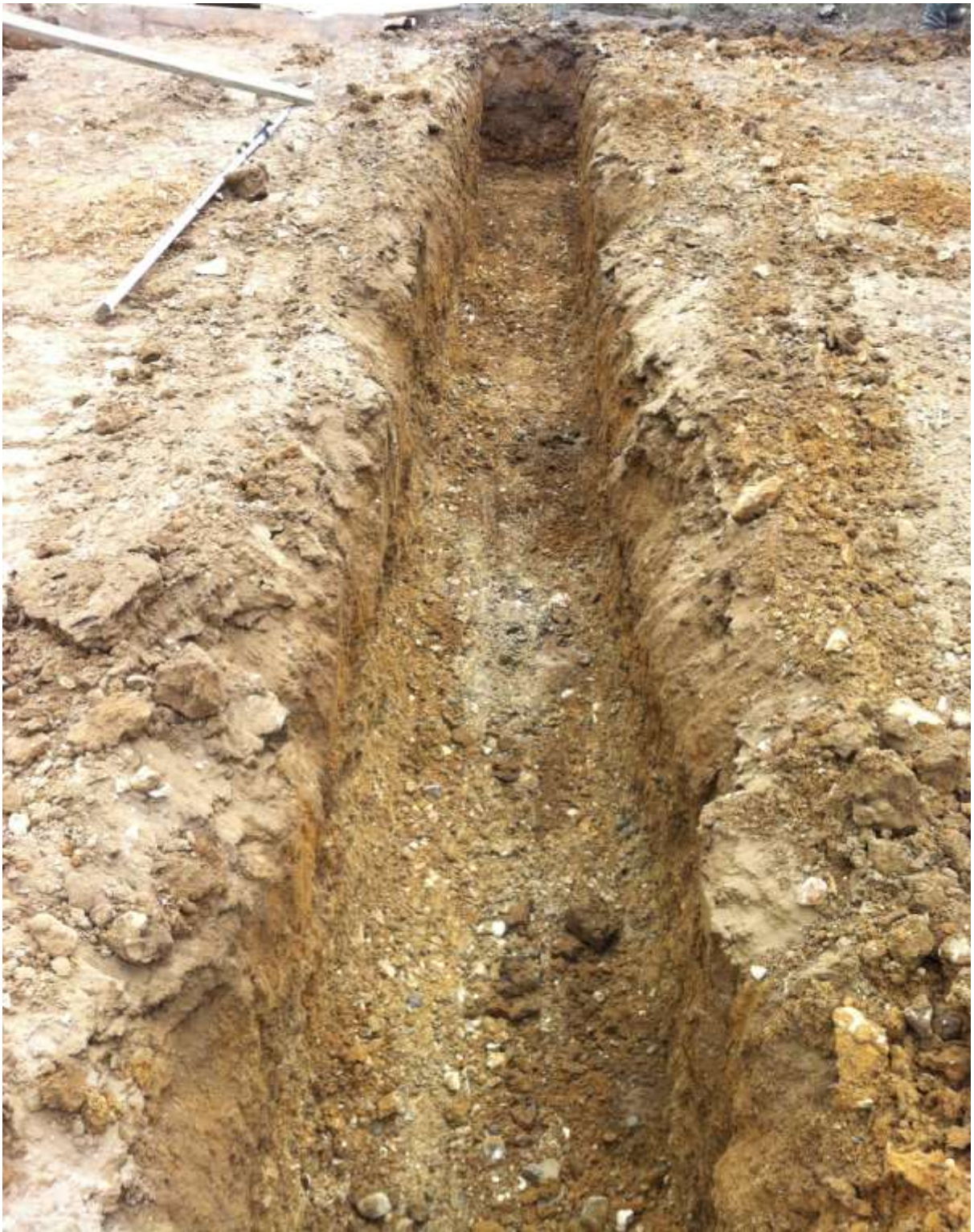
Plate 2. Close-up of foundation trenches
