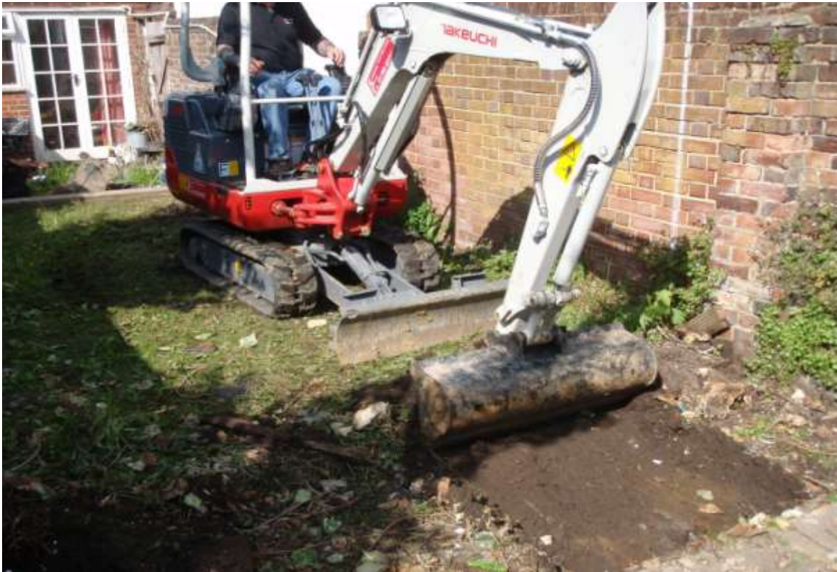
Plate 1 – Location of Trench 1 (looking SW)
