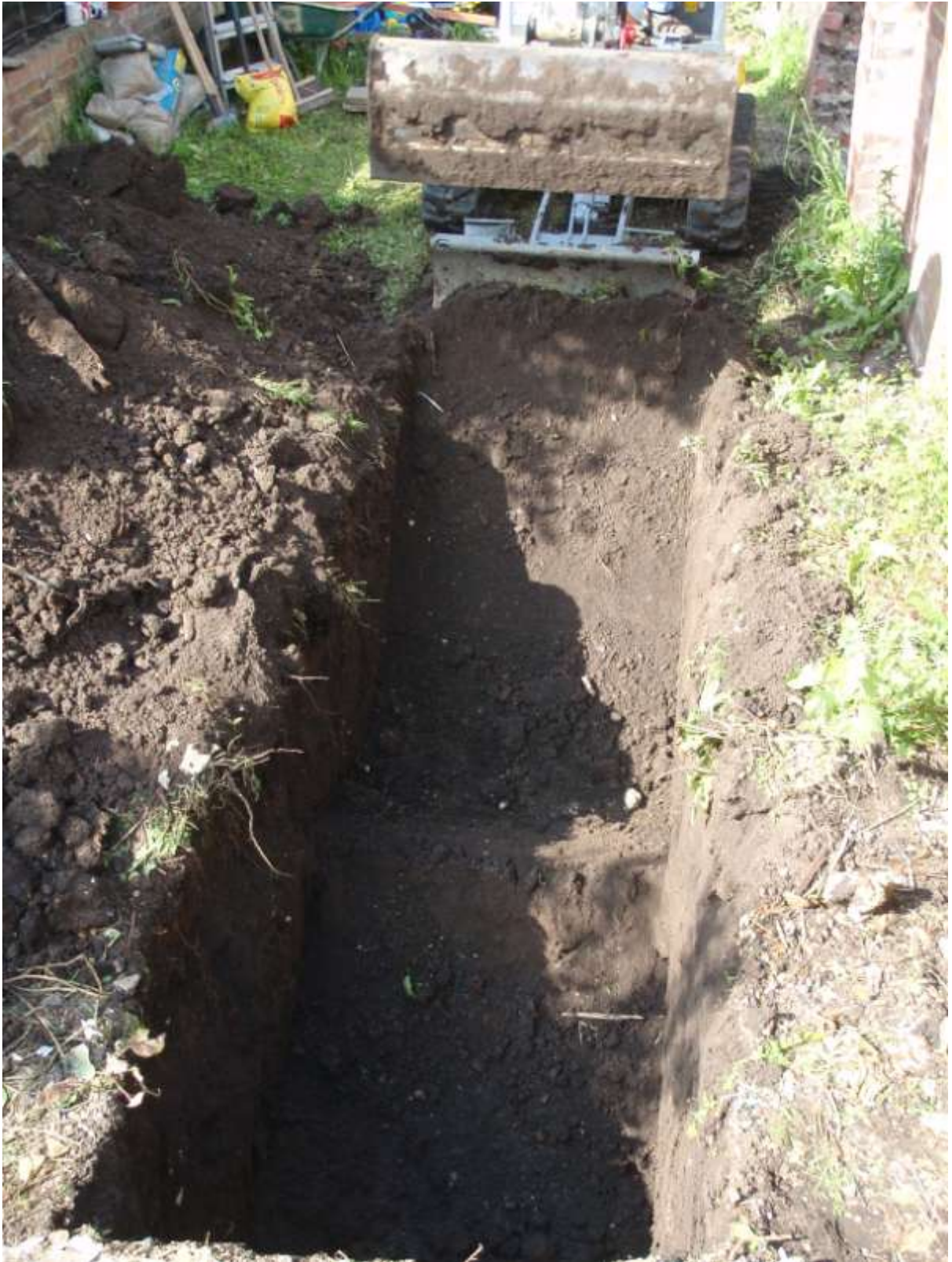
Plate 3 – Trench 1 being excavated (looking NE)
