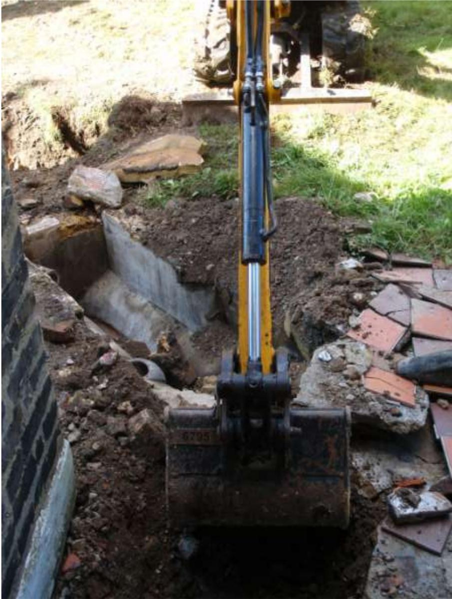
Plate 6. Cutting of the foundation trenches on south side
