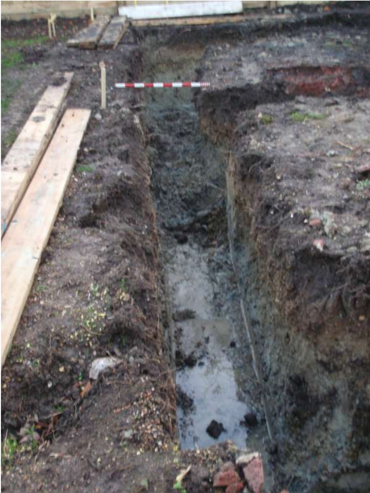
Plate 5. Foundation trenches on the east side
