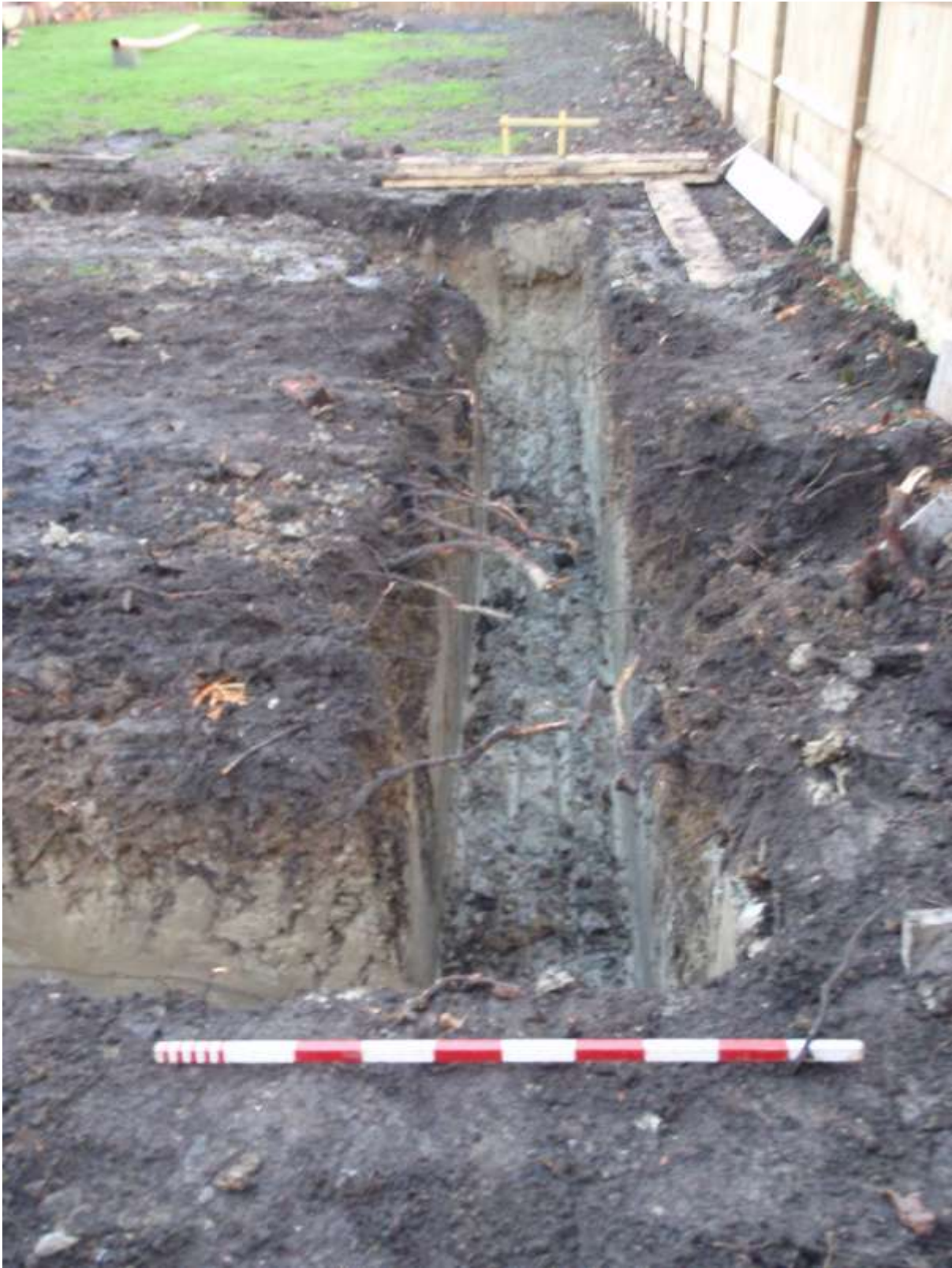
Plate 6. Foundation trenches on the south side
