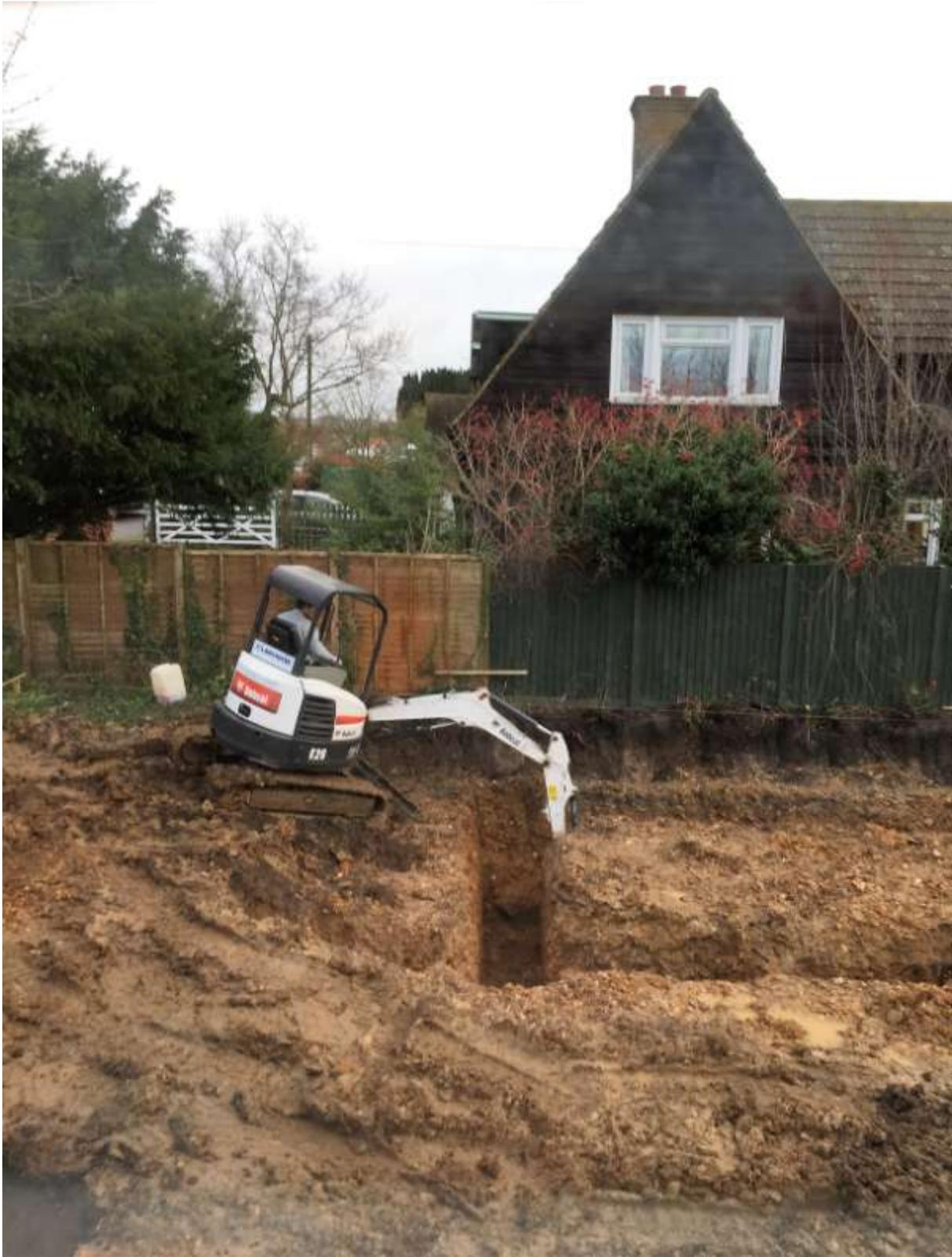
Plate 4. The site showing cutting of foundation trenches on the north-east side
