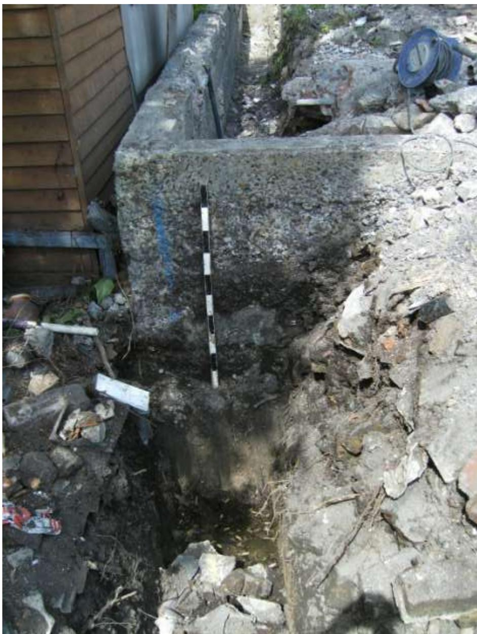
Plate 5. Depth of foundation trench
