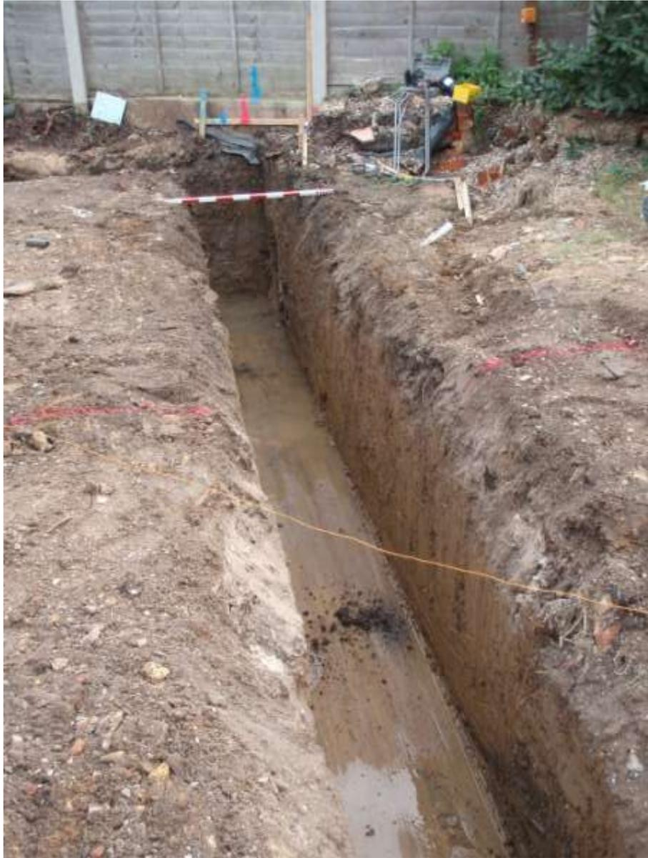
Plate 7. Cutting of the foundation trenches on the south side
