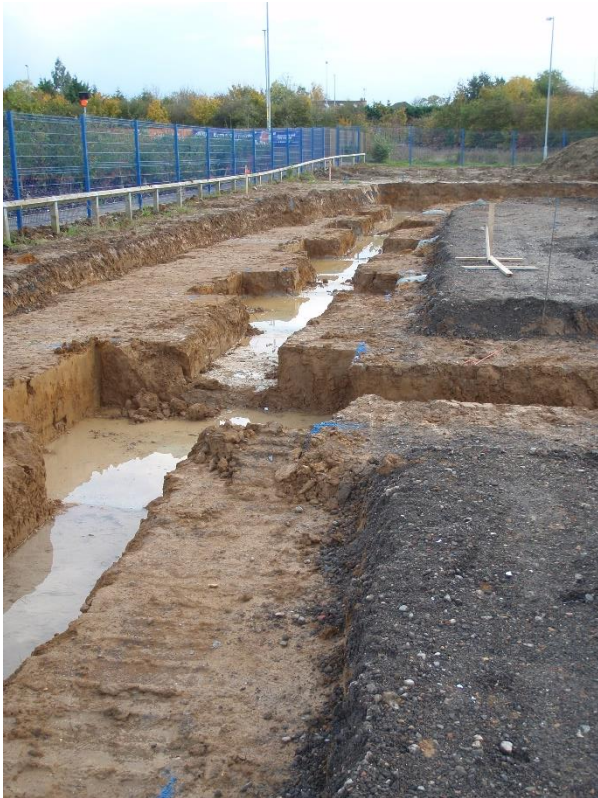
Plate 8. Completed foundation trenches (looking SSE)
