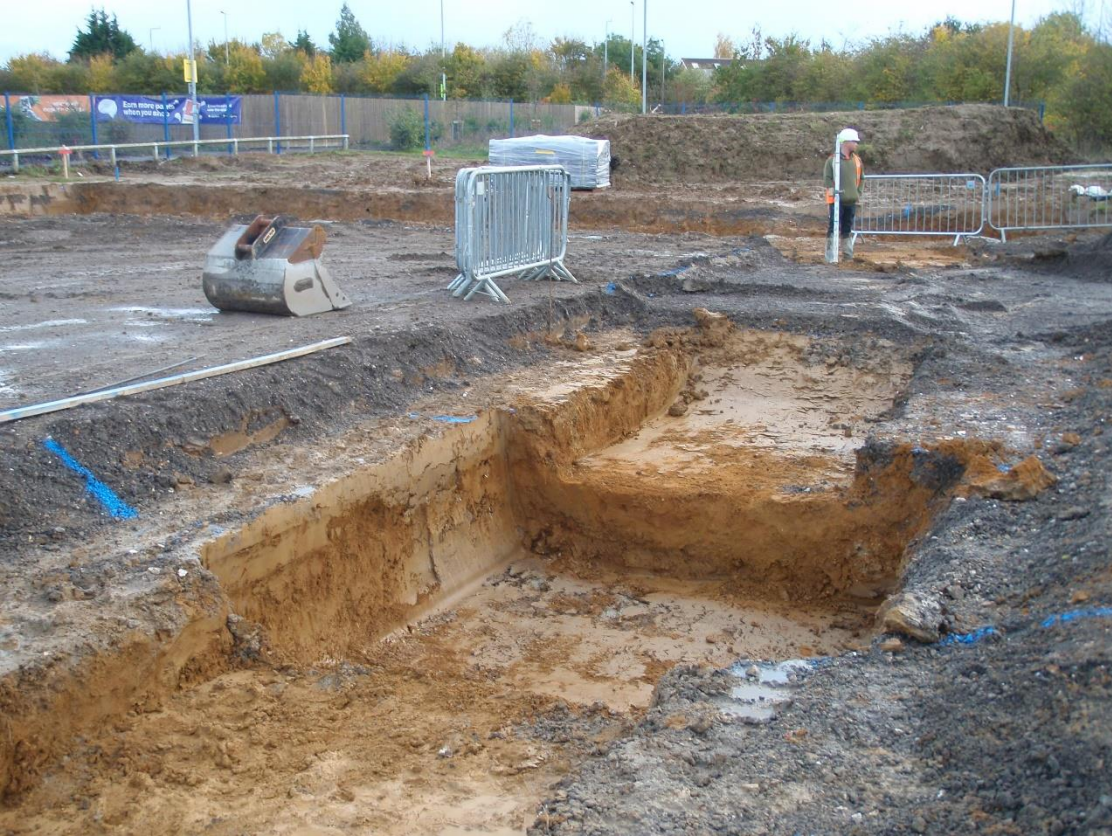
Plates 6. View of foundation trenches (looking NE)
