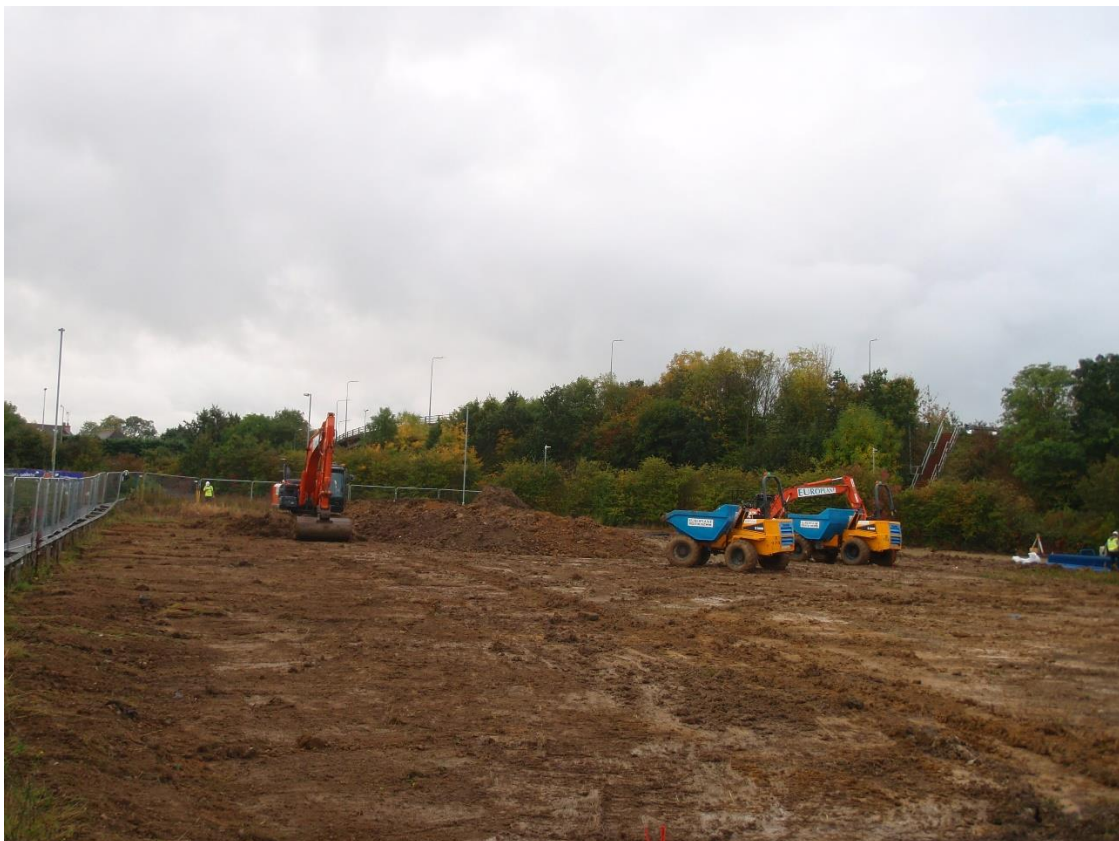
Plate 3. View of ground reduction (looking S)
