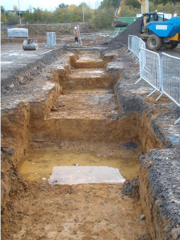
Plate 7. View of foundation trenches (looking E)
