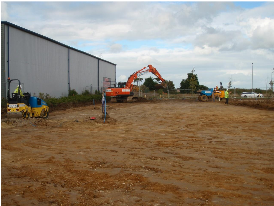
Plate 5. View of completed strip
