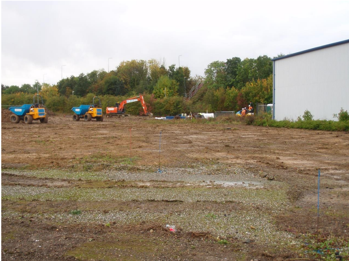
Plate 2. General view of site with topsoil strip (looking SW)
