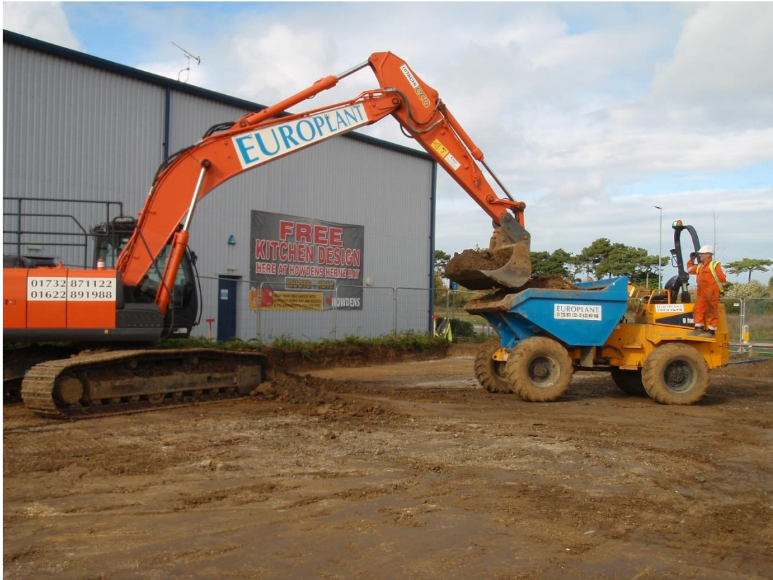
Plate 4. View of subsoil strip (looking NW)
