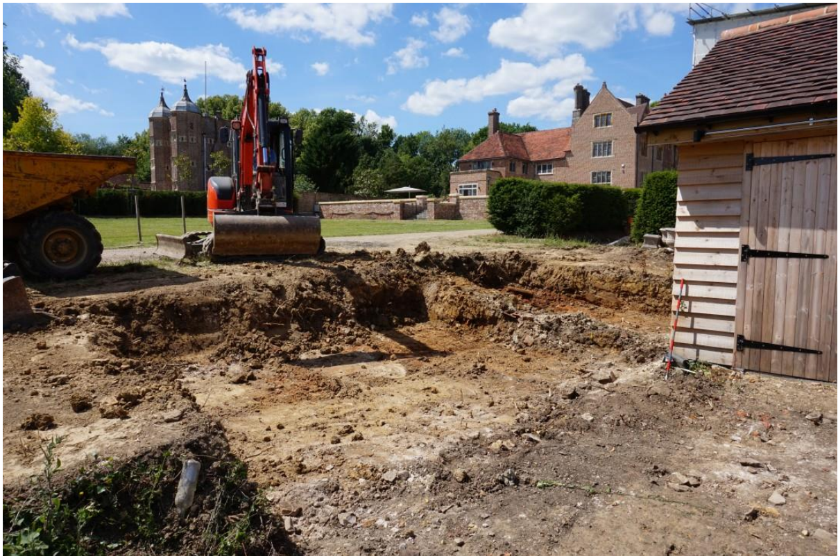
Plate 6: Levelling ground (Task 1)
