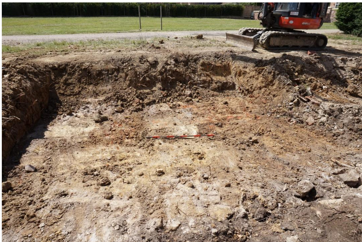
Plate 5: Looking west at ground reduction (Task 1)
