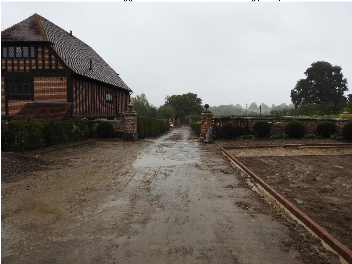
Plate 11: Removal of tarmac prior to re-instatement (Task 4)
