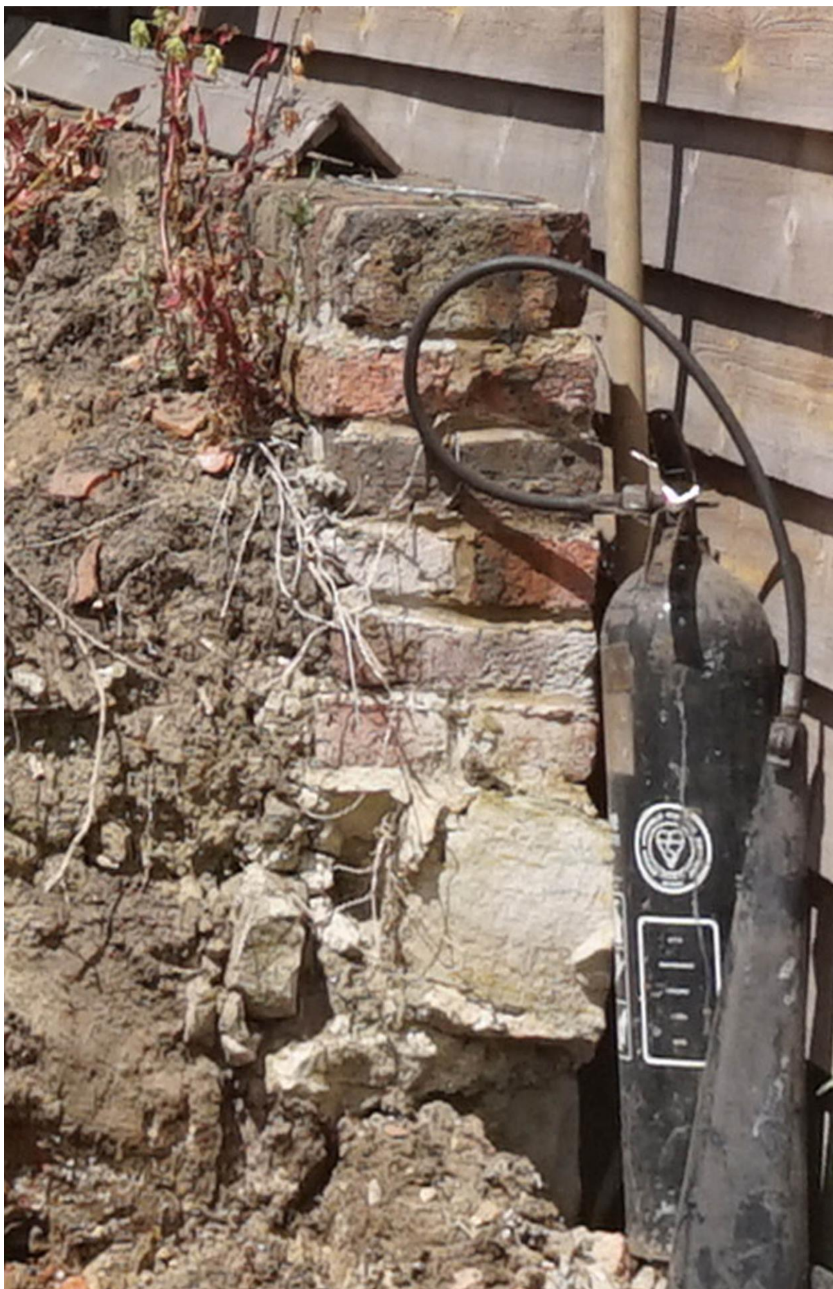
Plate 13: Retaining wall I (105) exposed in section on northern wall of trench 1. Lower part was constructed of dressed sandstone
