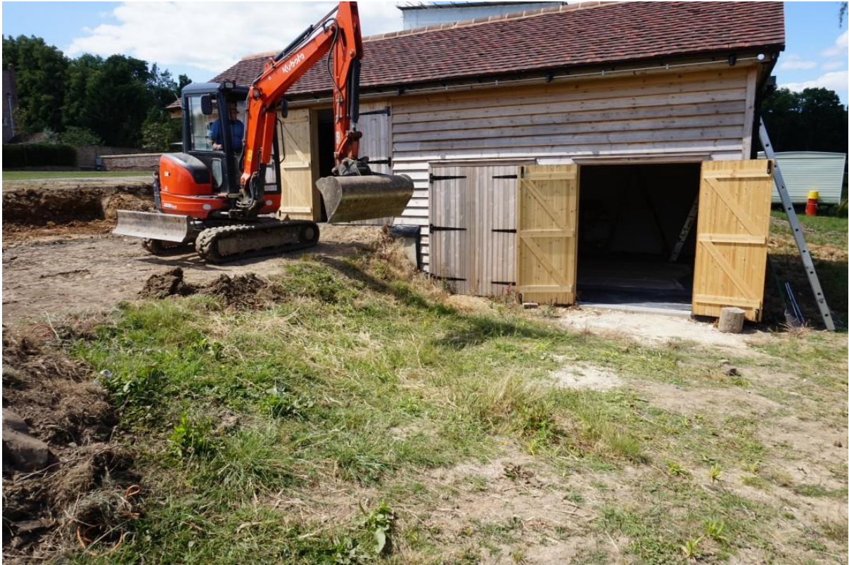
Plate 8: Looking north prior excavation of foundation trenches (Task 2)
