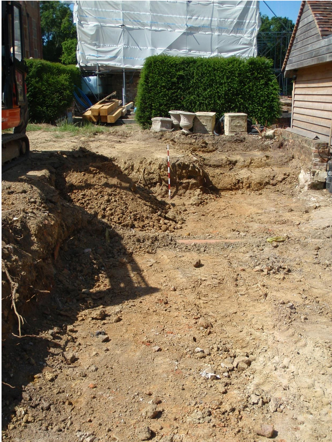
Plate 3: Looking east at excavation of retaining wall area (Task 1)
