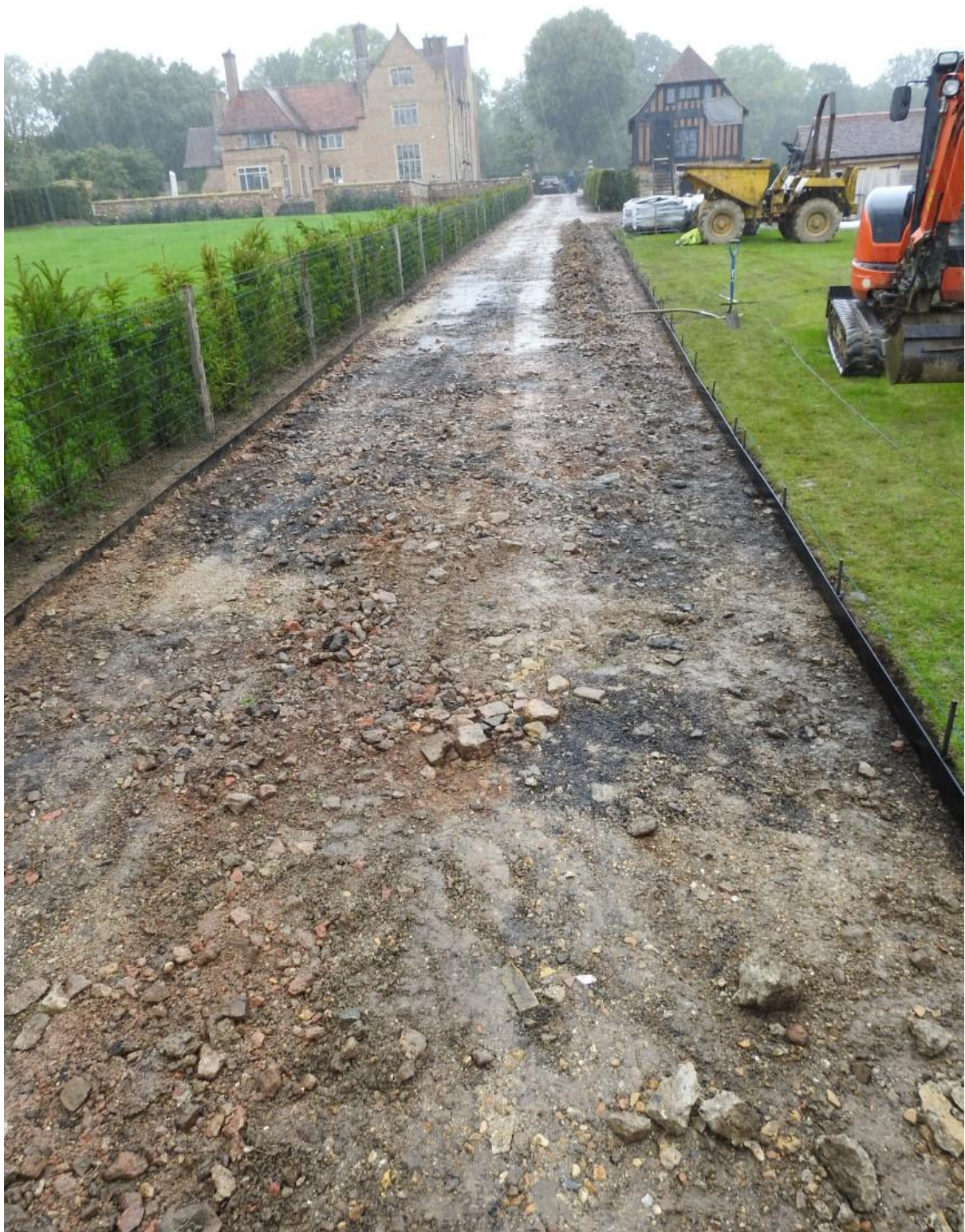
Plate 12: Removal of tarmac (Task 4)
