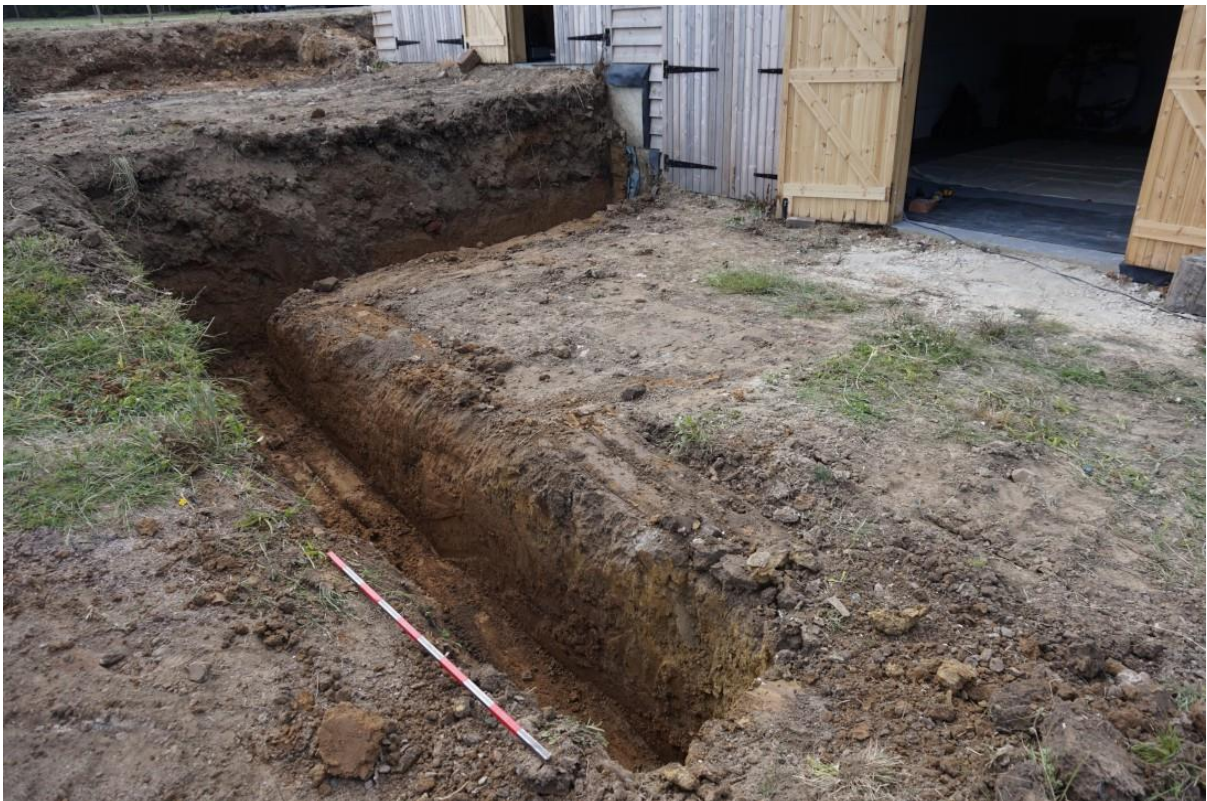
Plate 9: Looking north west at foundation trenches (Task 2)
