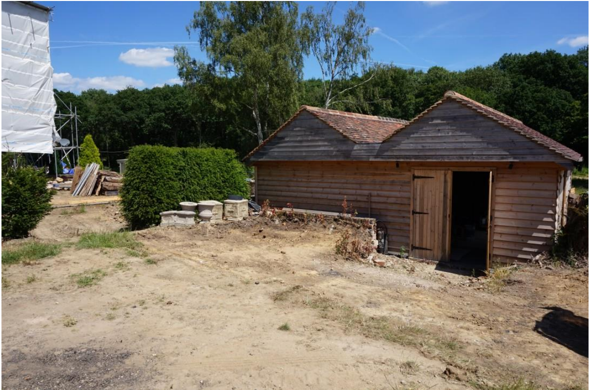
Plate 1: Looking NE at the area of ground to be lowered (Task 1)
