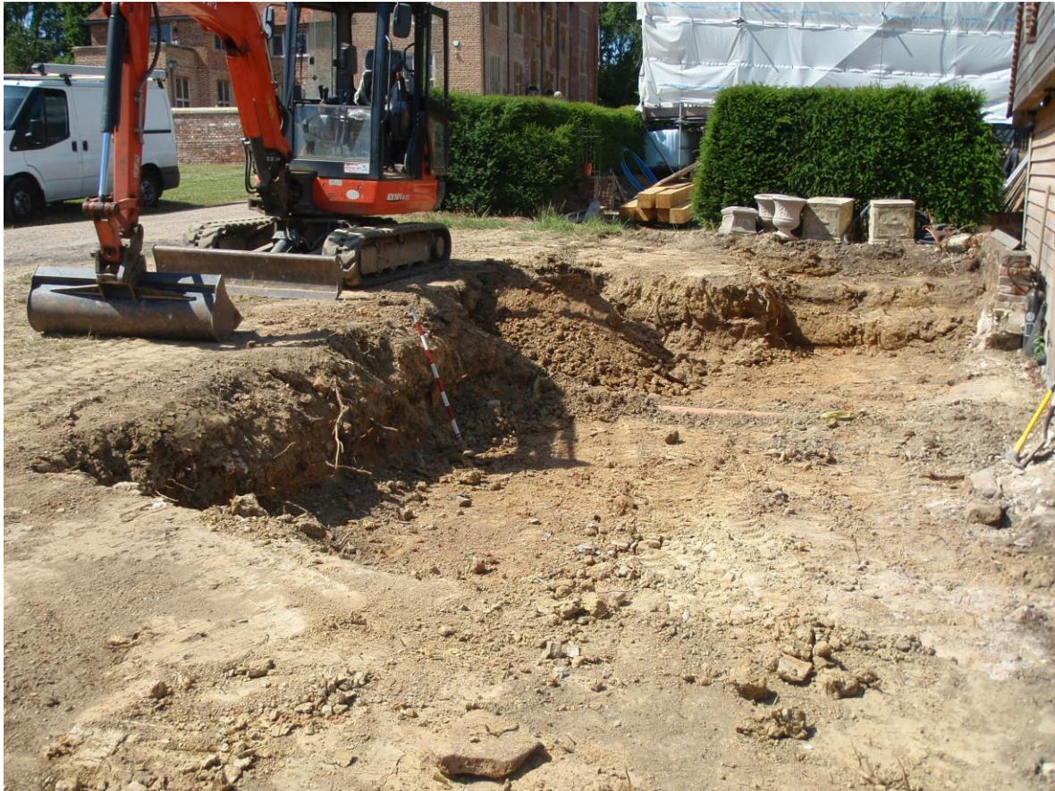
Plate 10: Levelling ground west and south of the outbuilding (Task 3)
