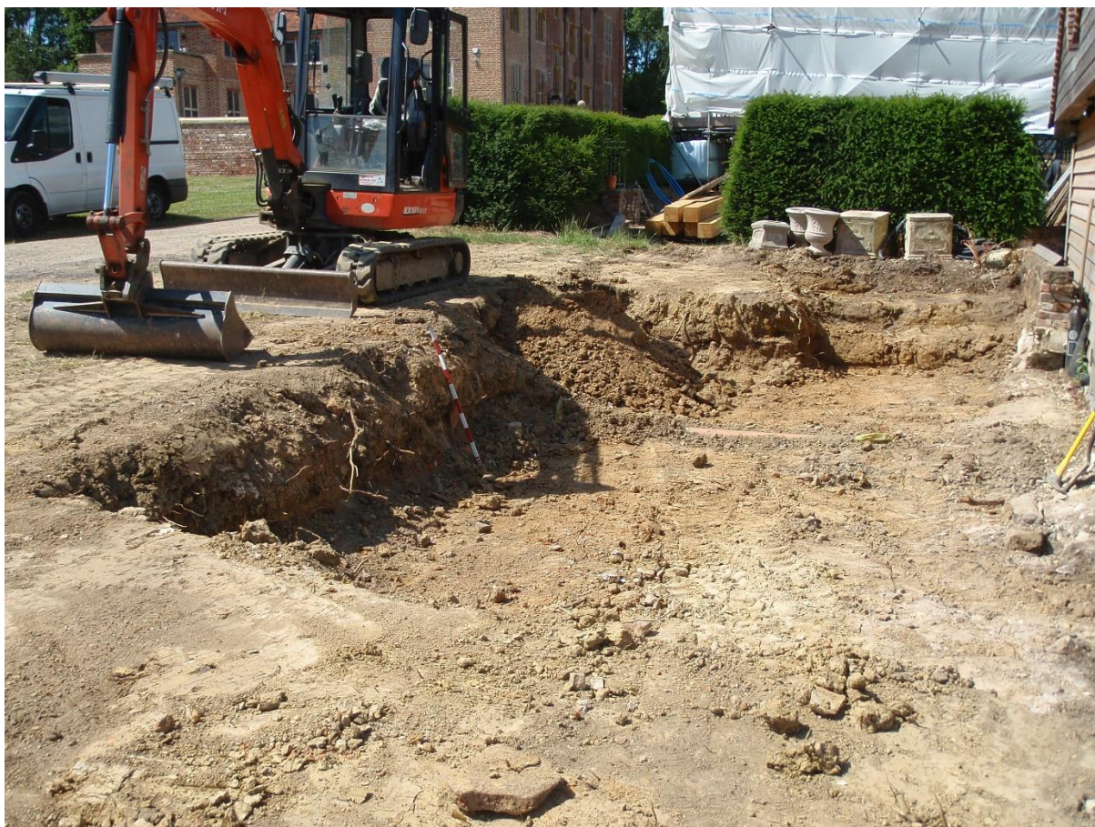
Plate 4: Looking north at ground reduction (Task 1)
