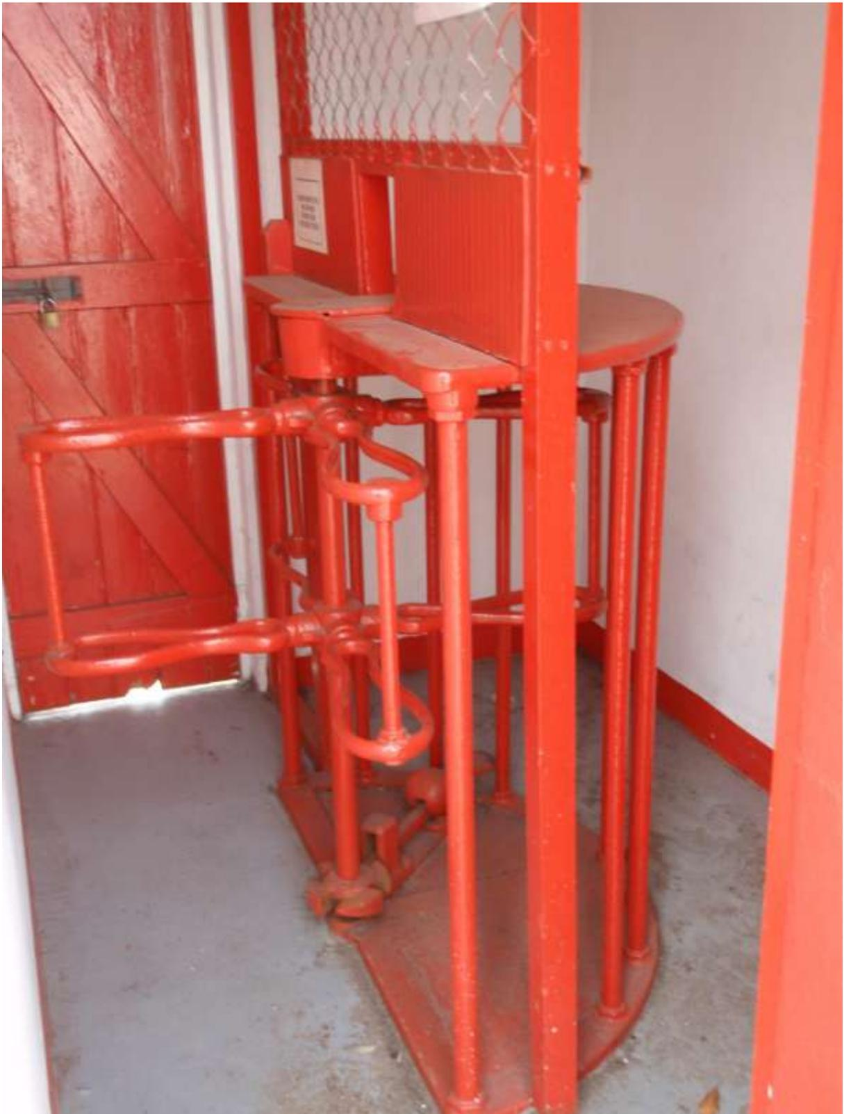
Plate 16. Detail of the turnstile inside the entrance gates
