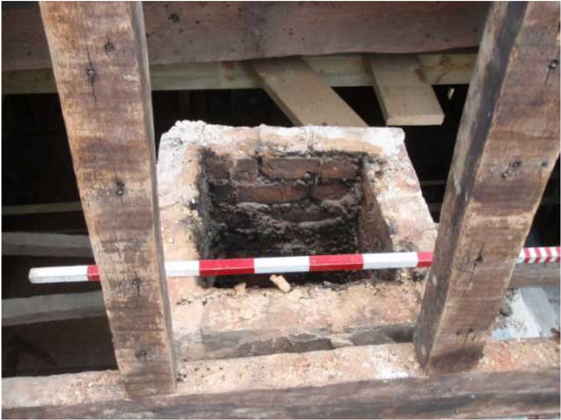
Plate 11. Chimney flue
