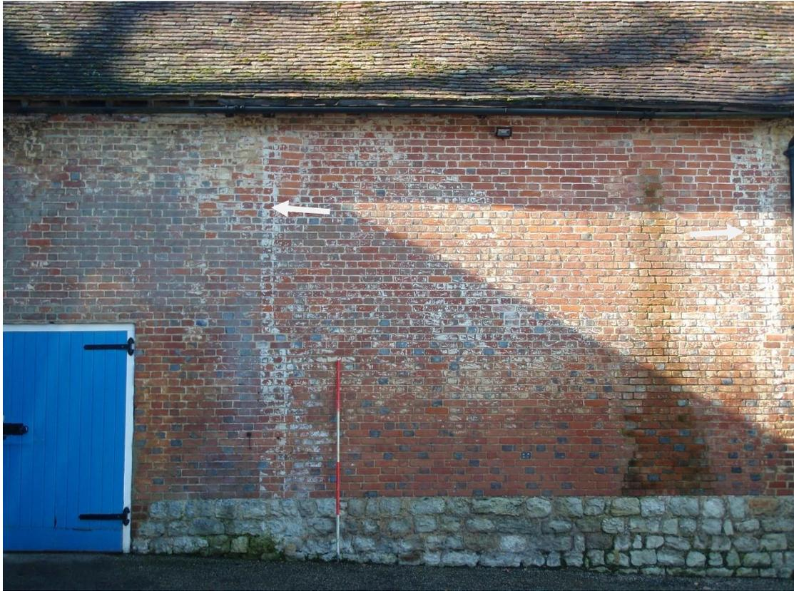
Plate 7. View of east facing frontage (Note build mark of demolished extension)
