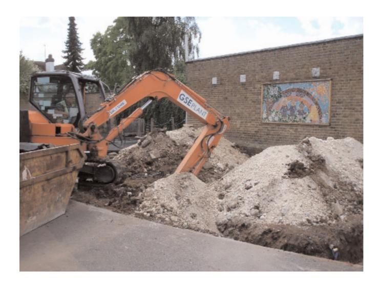
**Plate 1.** Location of site of proposed development at Ethelbert Primary School, Ethelbert Road, Faversham, Kent. (NGR 601054 160755). Facing south west with tarmac removed and foundation trenches being cut under archaeological supervision.
