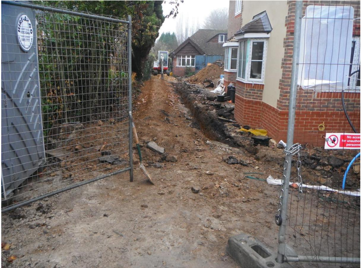
Photograph 2: Service trench (gas and water) (looking North West)
