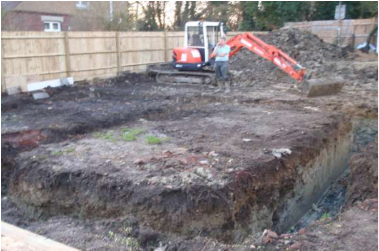
Plate 2. General view of site looking north-east
