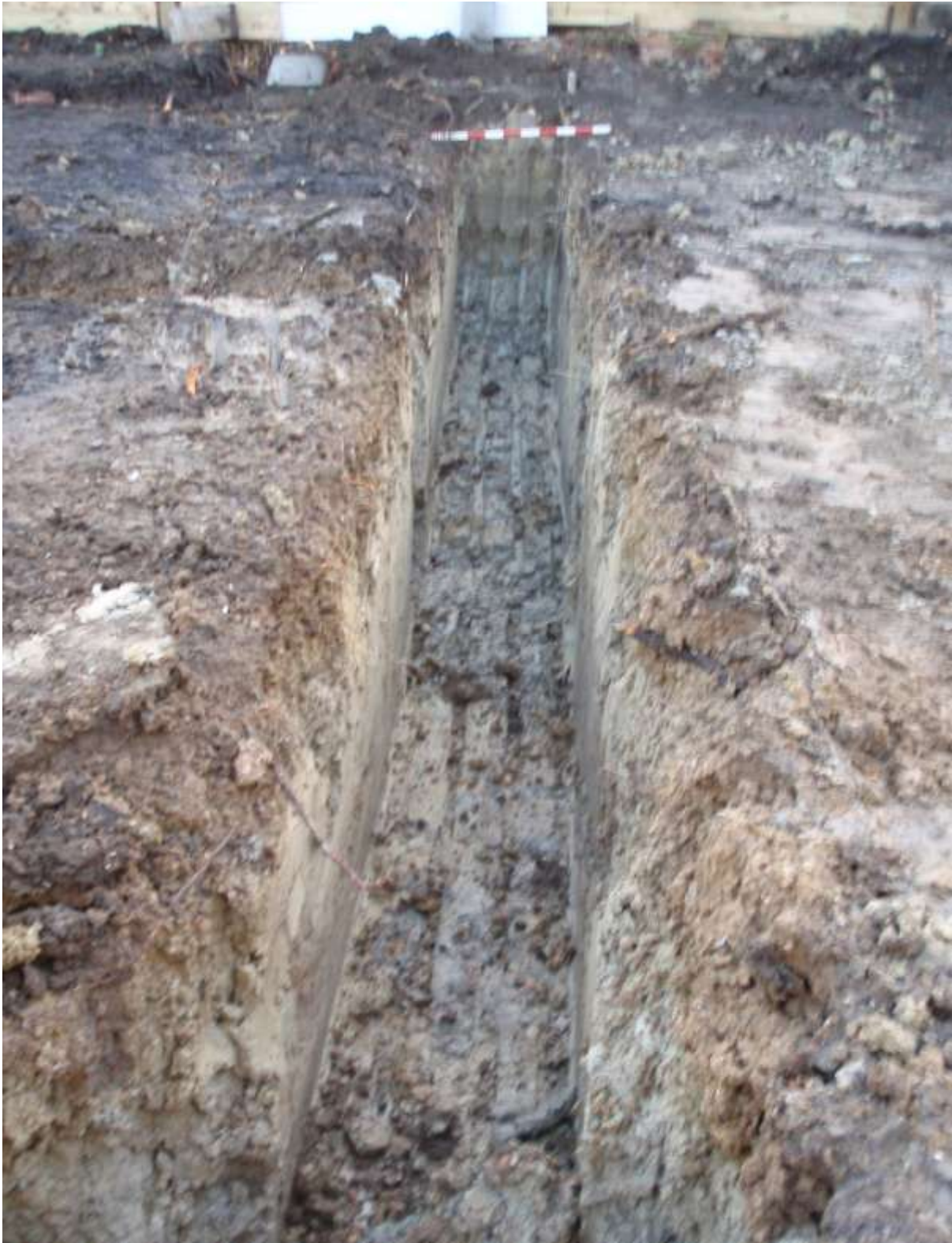
Plate 4. The site showing cutting of foundation trenches on the west side
