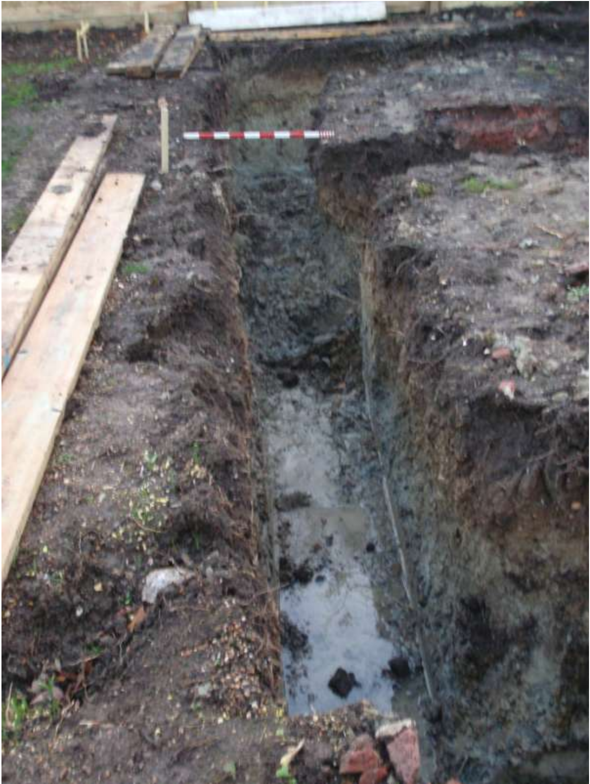
Plate 5. Foundation trenches on the east side
