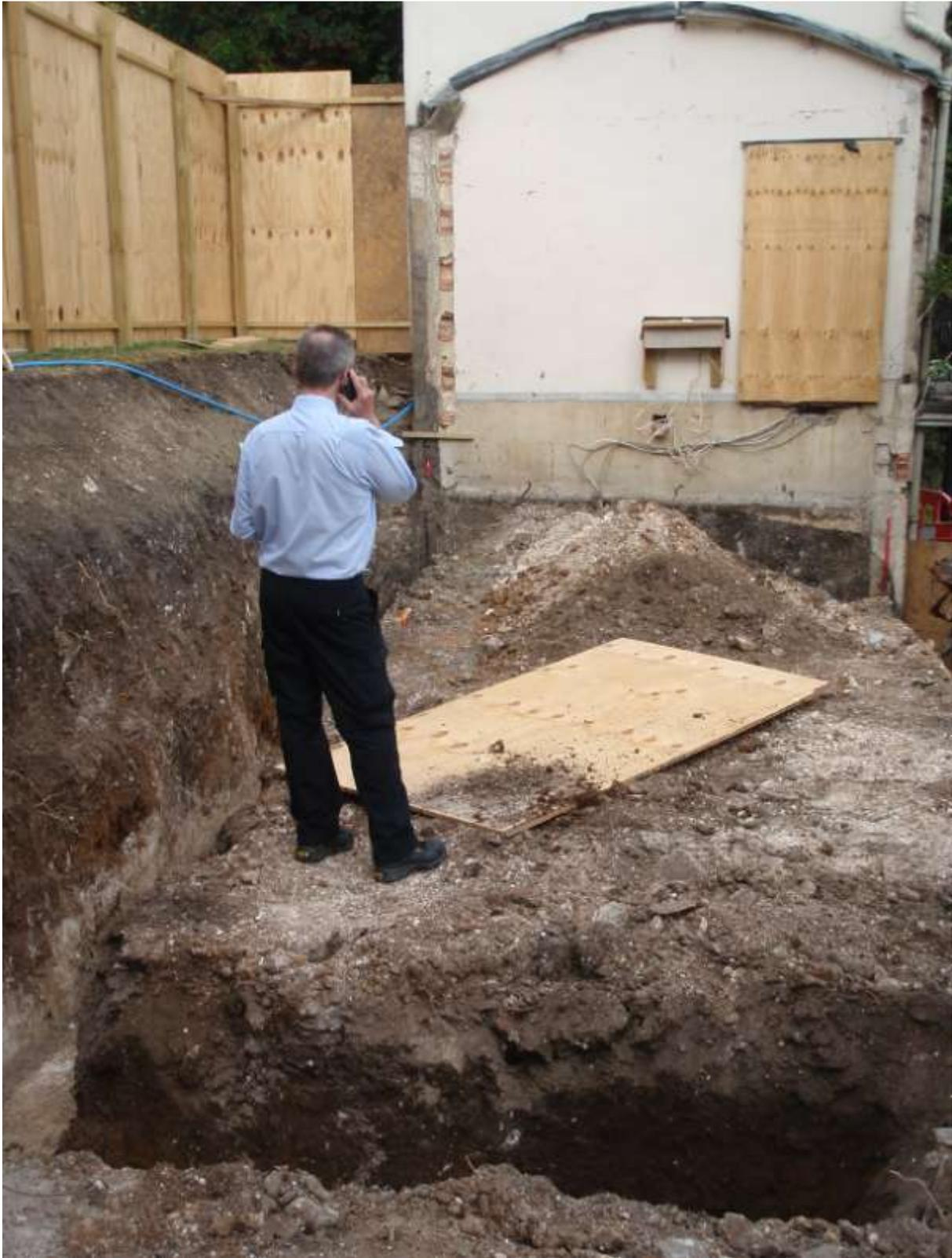
Plate 5. Foundation trenches completed
