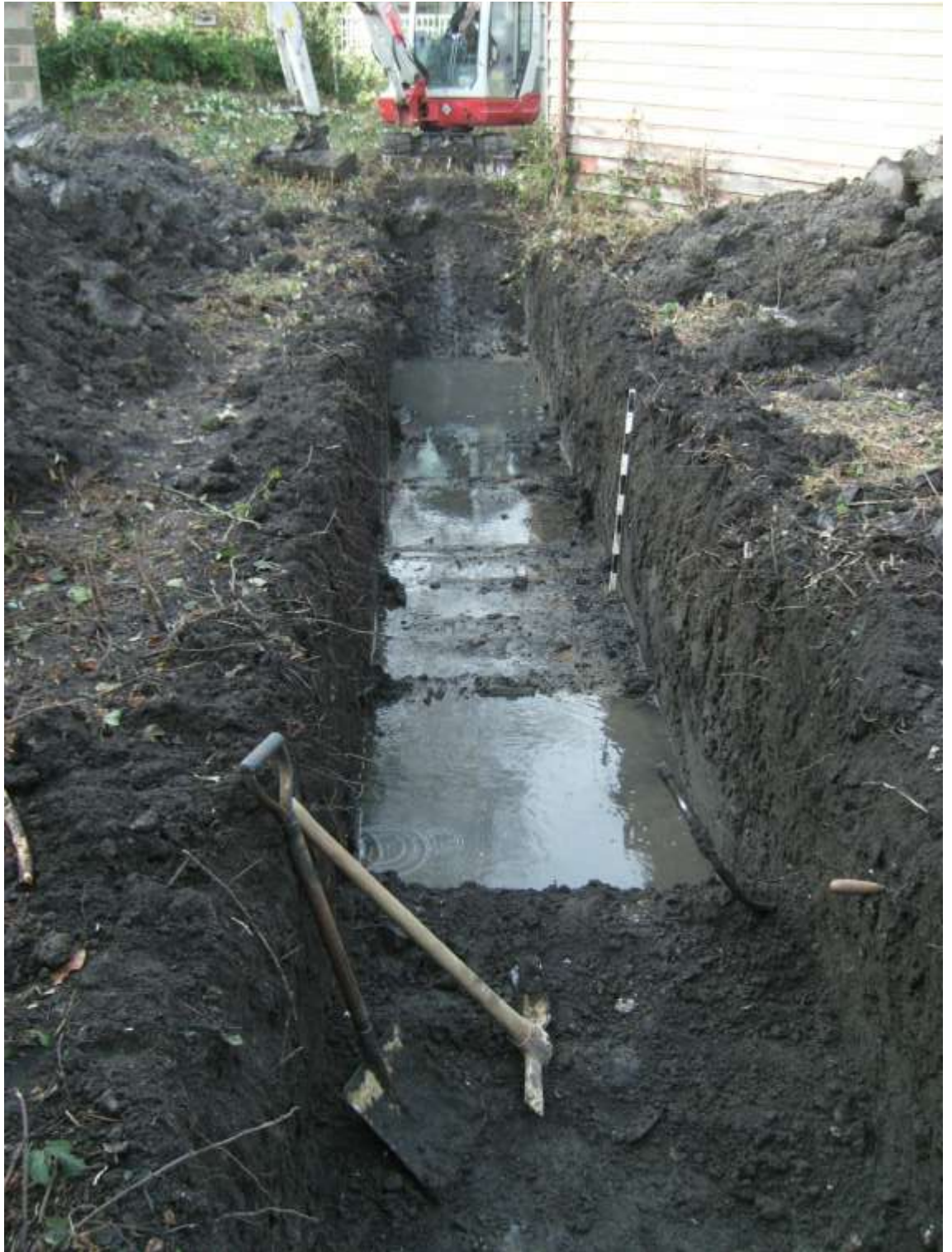
Plate 5. Excavated trench (looking NNW)
