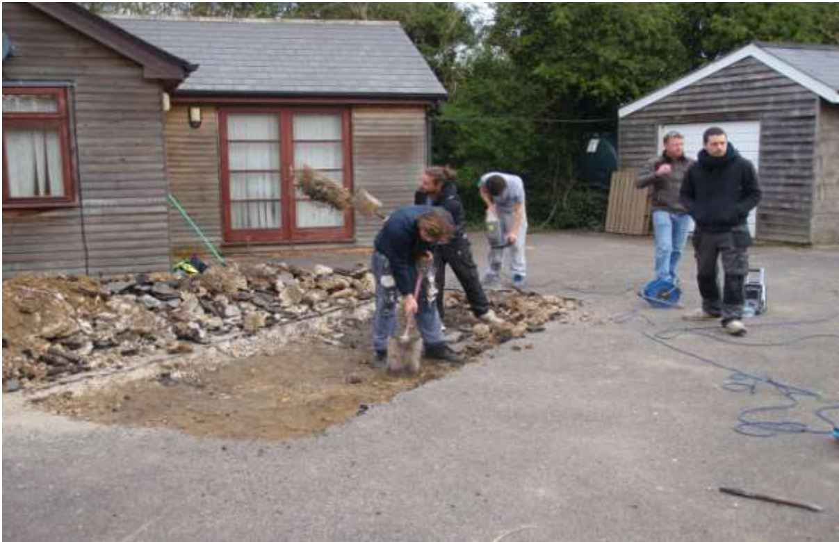
Plate 1 – Location of Trench 1- breaking out concrete (looking NW)
