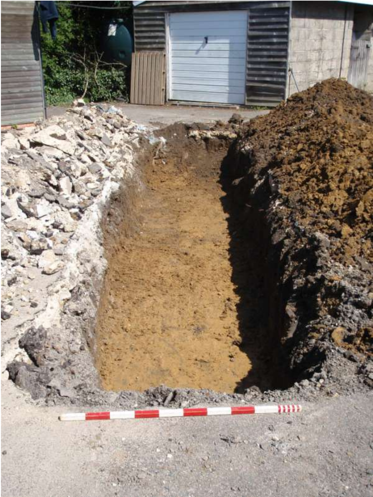
Plate 5- Trench 1 (looking N)
