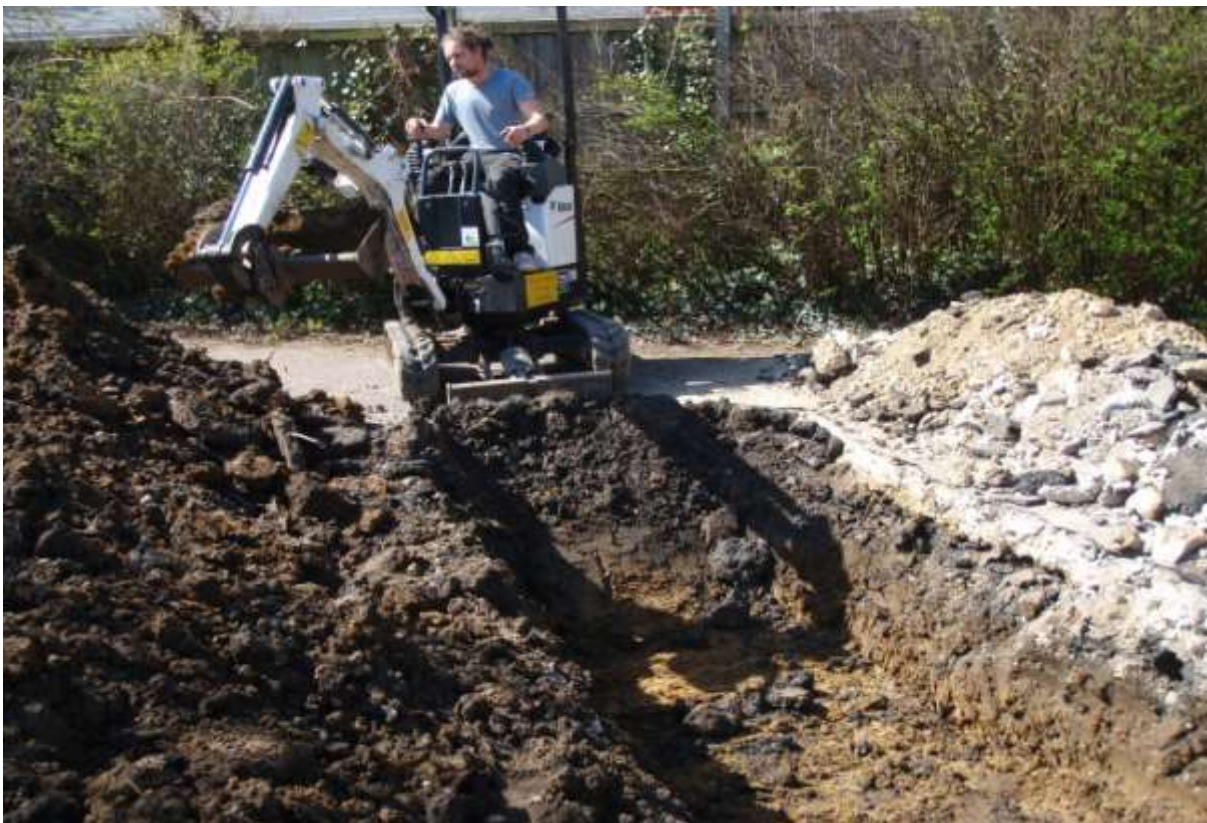
Plate 2 –Trench 1. Mechanical excavation (looking S)
