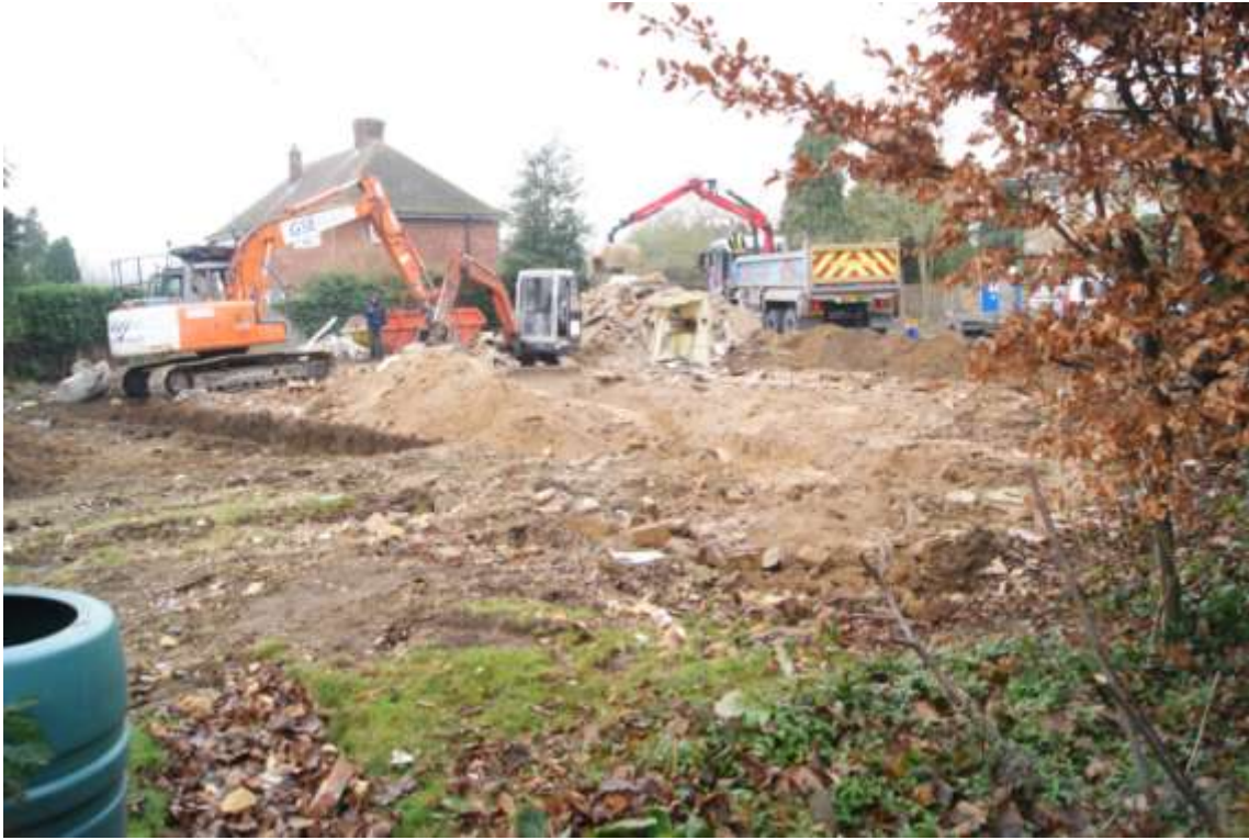
Plate 2. View of site (looking north)
