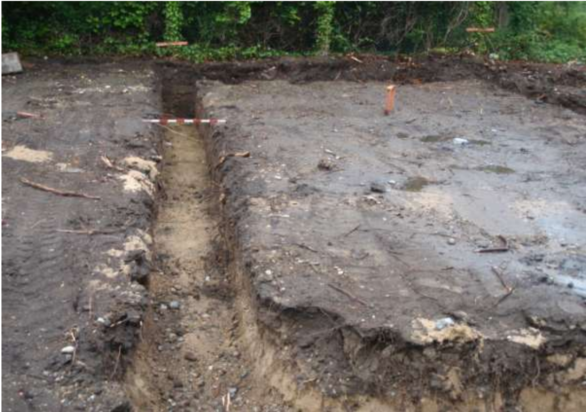
Plate 6. View of foundation trenches on the east side
