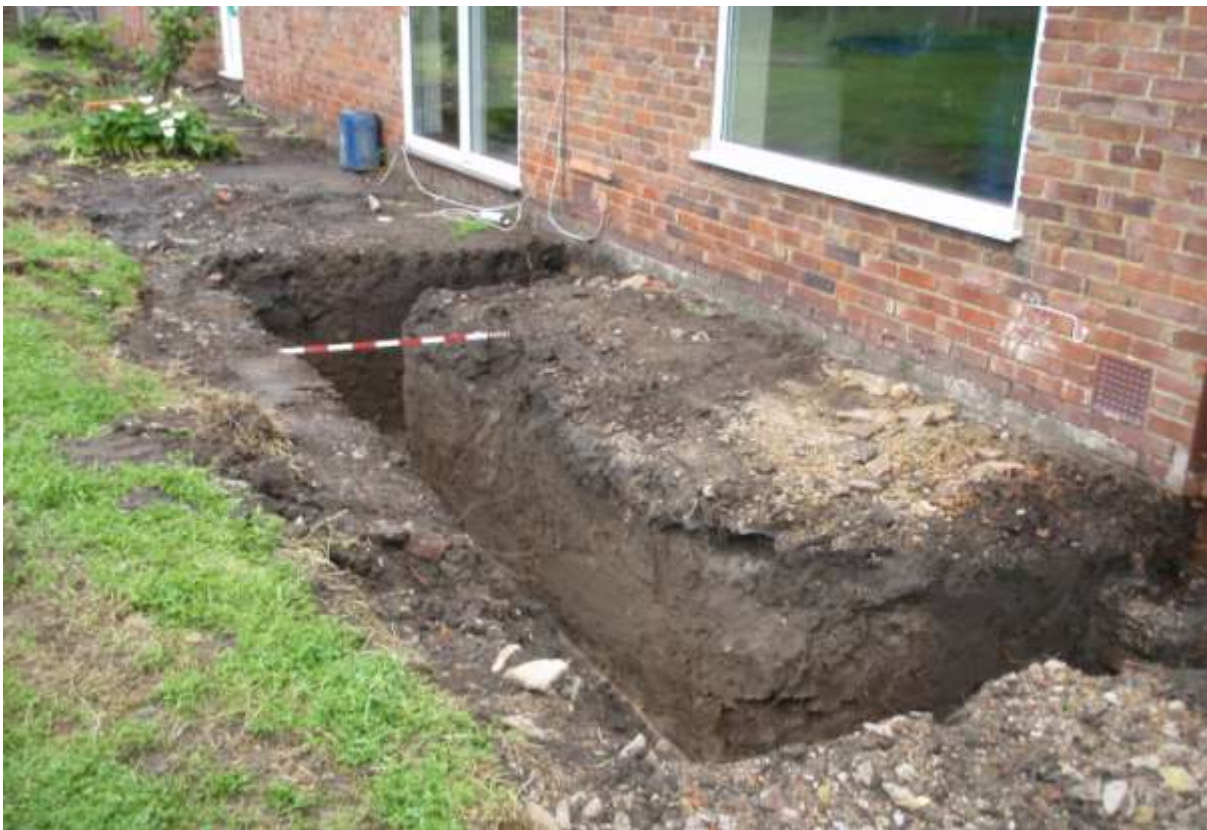
Plate 5. Foundation trenches on the south side
