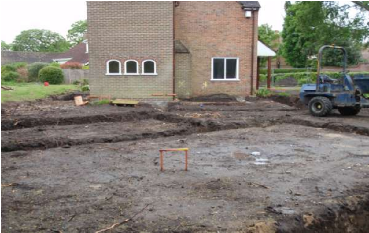
Plate 4. The site showing cutting of foundation trenches on the east side
