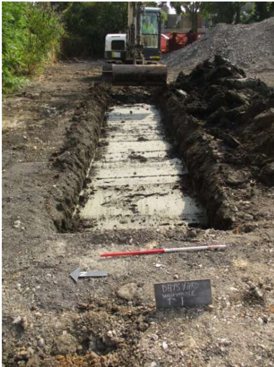
Plate 2. Trench 1 (looking NE)
