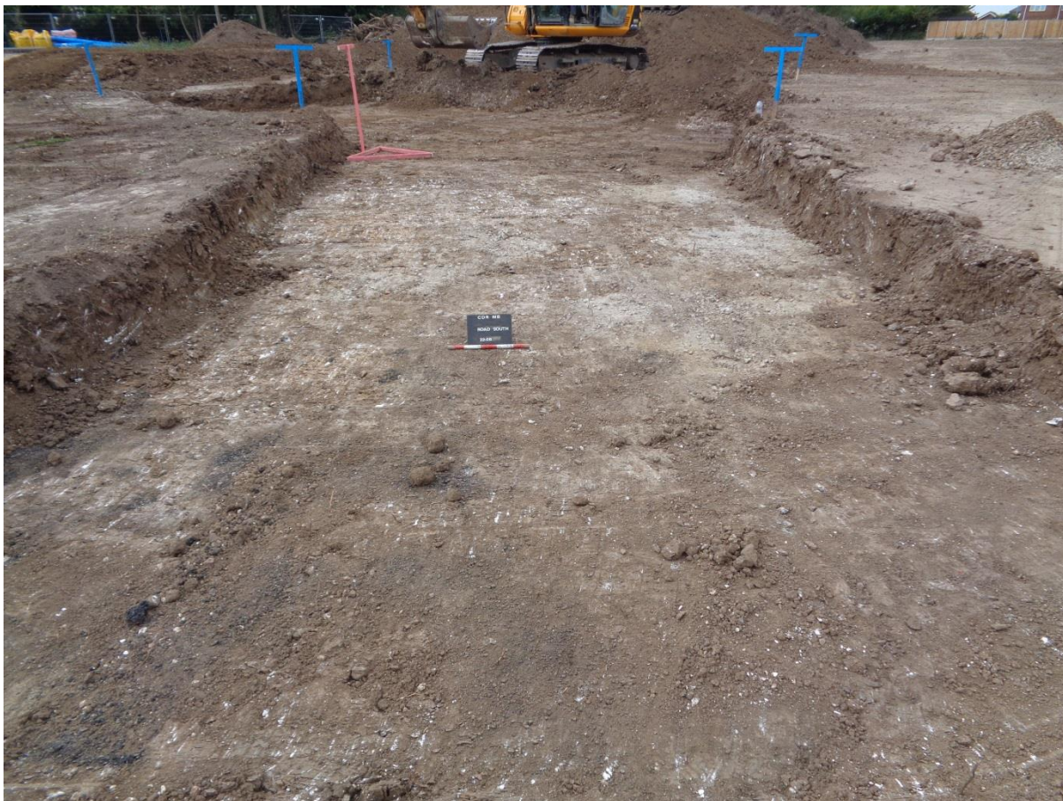
Plate 2. General view of the depth of road strip and house platform strips.
