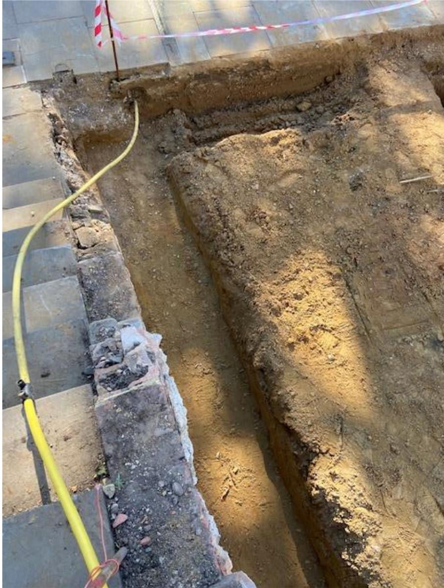
Plate 7. View of site reduction and stepped foundations
