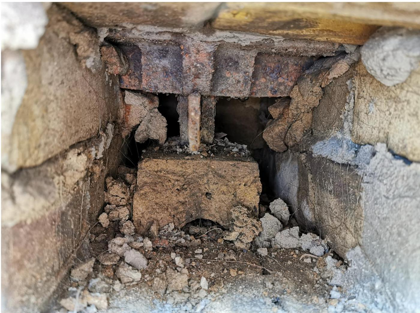
Plate 22: Leaver mechanism in located inside the structure [1509]. It was turning vertical axle visible at the top of the structure.
