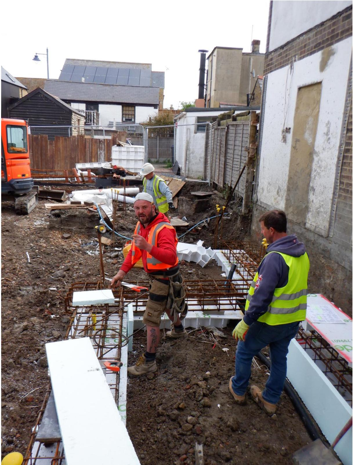
Plate 1. General view of site with formwork for concrete foundations (looking NE)
