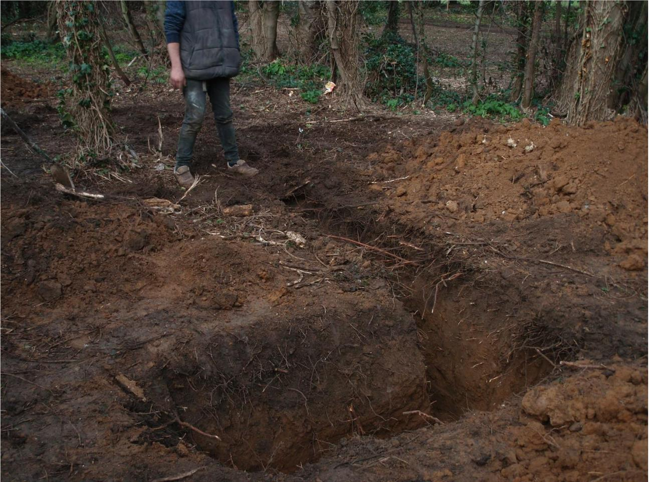
Plate 4. Trial Pit 1 being excavated
